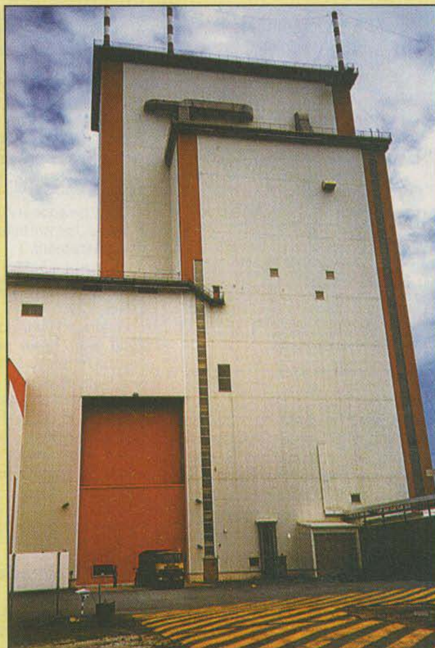
Phase 3-D's new, and hopefully temporary, home at the European Space Agency's launch facility in French Guiana. If you look very carefully at the bottom, you may be able to see the truck delivering the P3D satellite. (Photo by Peter Gülzow, DB2OS, courtesy AMSAT-DL)
