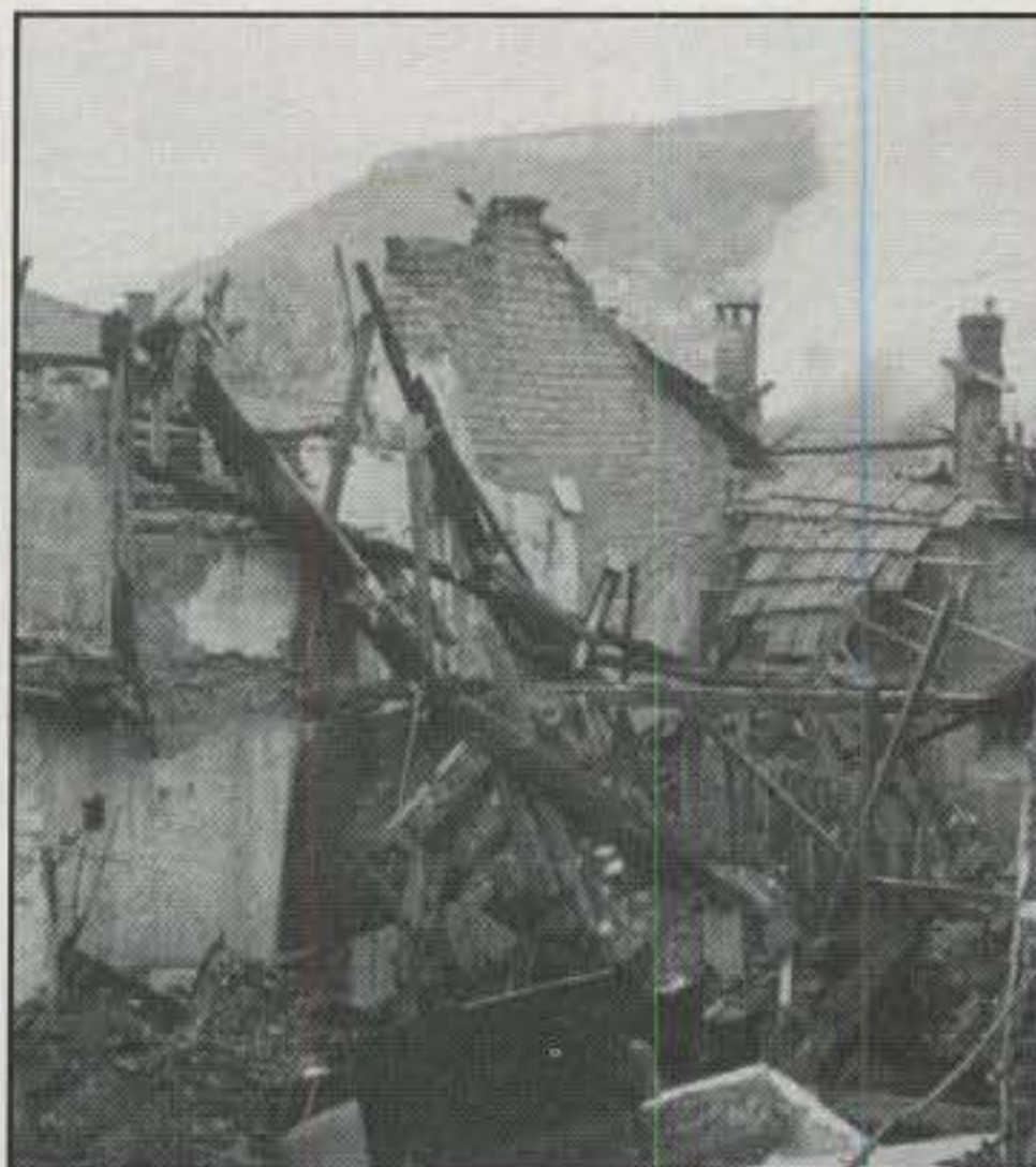
These destroyed buildings are across the street from the Caritas headquarters in Prizren. "There are no words to describe this," said Marcos, IK5BHN. (Photos of Kosovo by IK5BHN)
