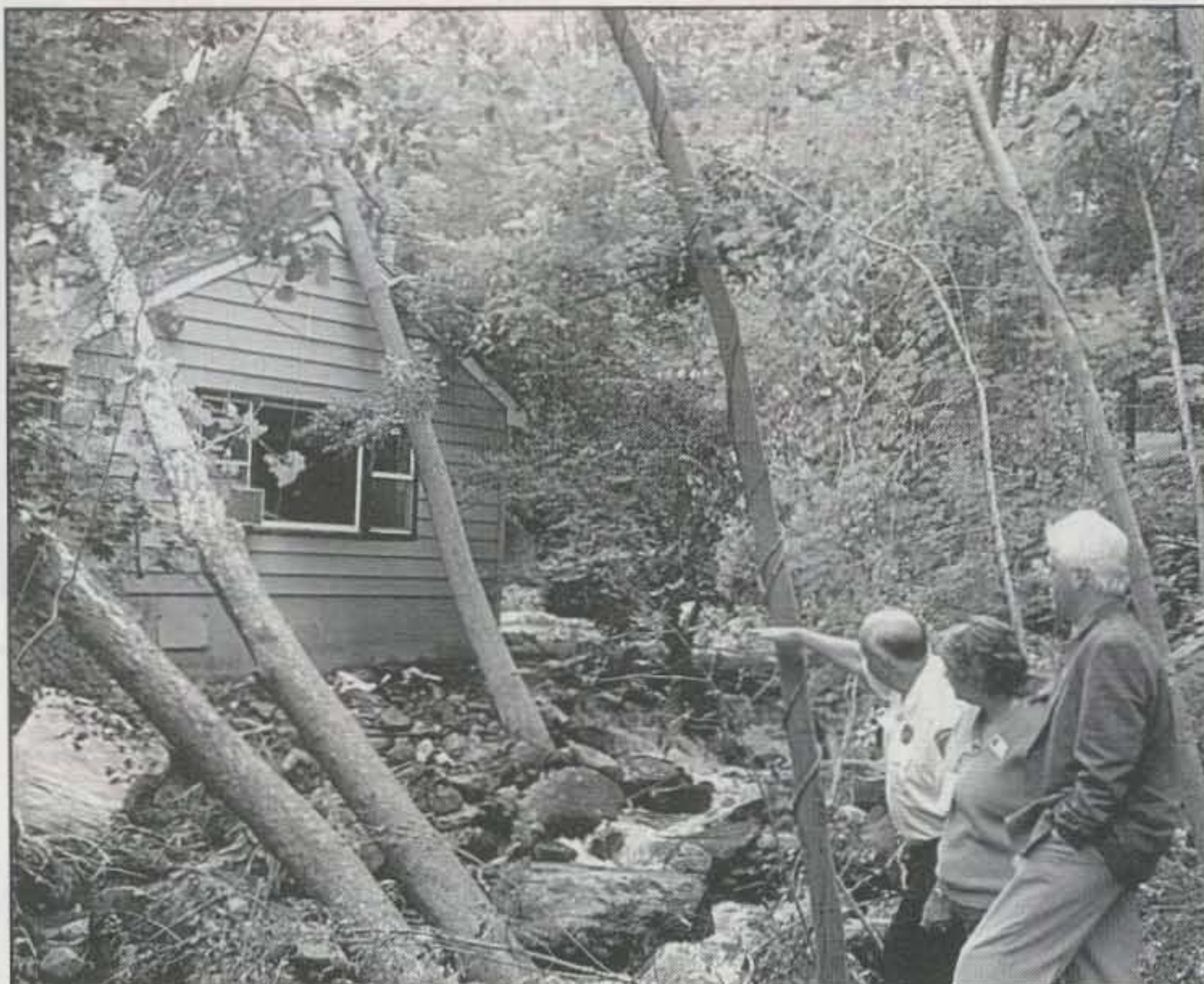
Heavy rains uproot trees onto local homes. Skip Danielson, County Emergency Management Director; Deb McKay, N2TTP, Skywarn Coordinator; and Jim Eberwine from the National Weather Service survey the damage. (Photo courtesy Deb McKay, N2TTP)
