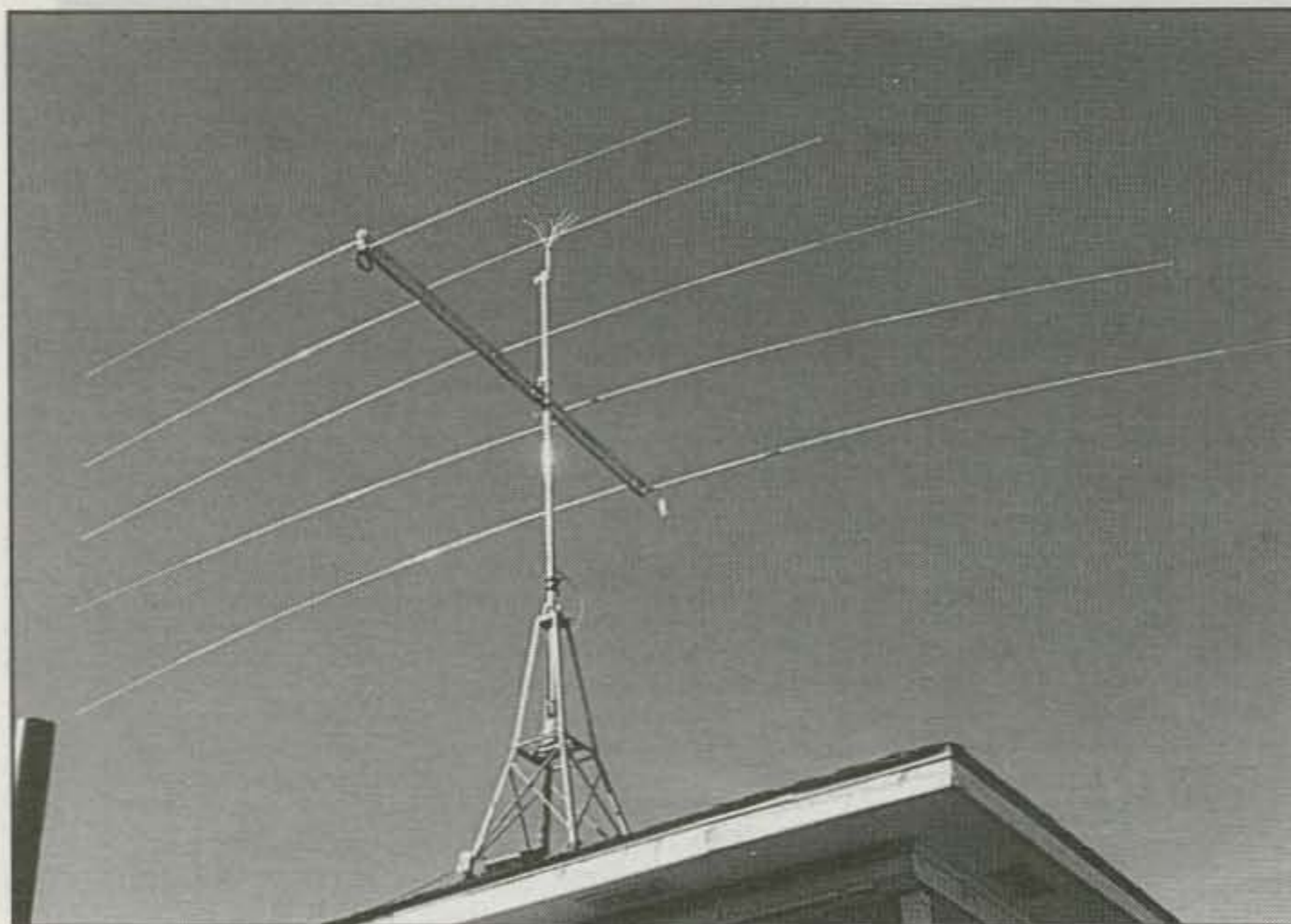
A roof tower is an acceptable compromise when circumstances dictate its use. A major drawback is that it brings the antenna in close proximity to the house wiring located just beneath the roof.
