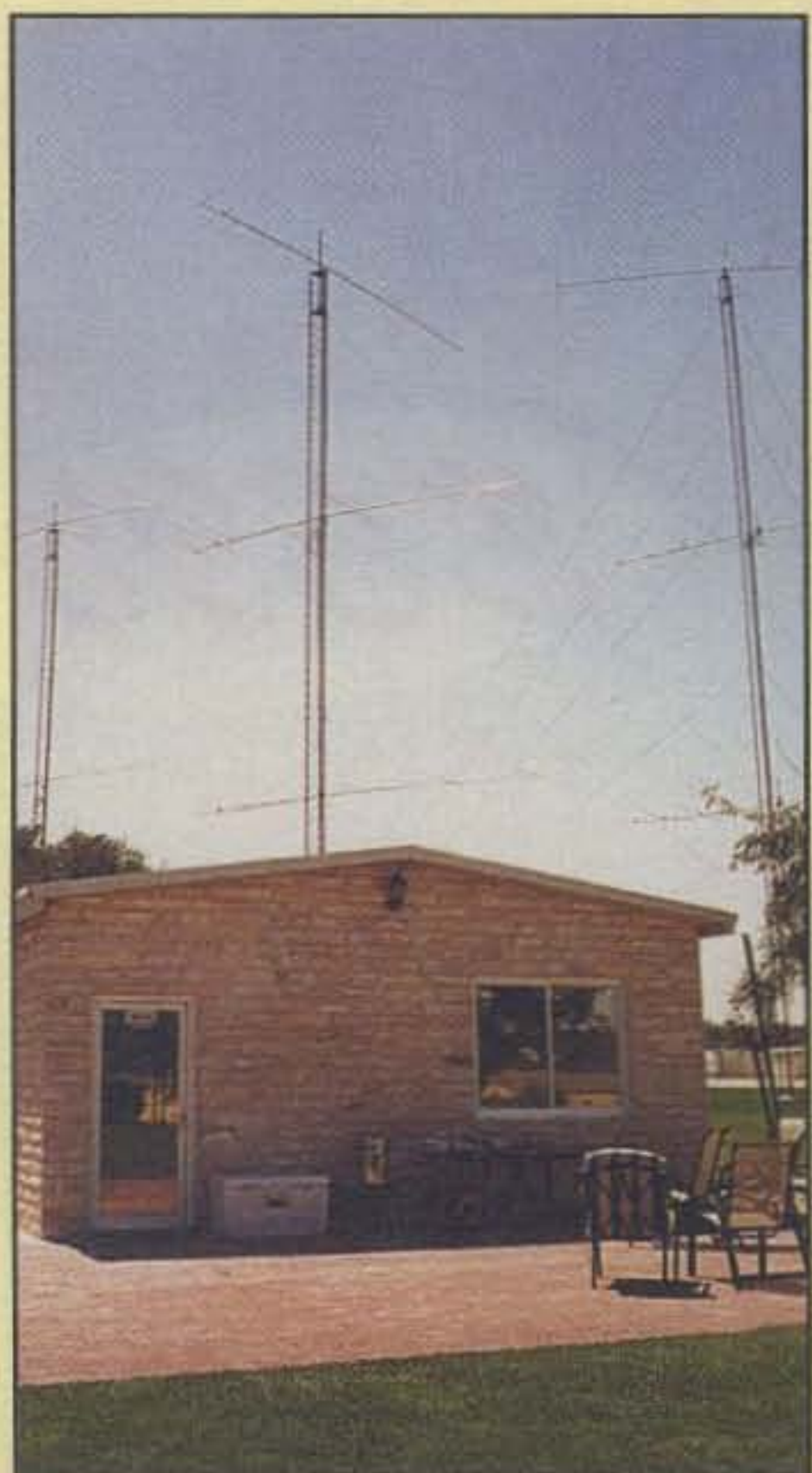
The building that houses the station was built in a record ten days just before the 1997 CQ WW DX CW Contest. (Photo by K2RED)
