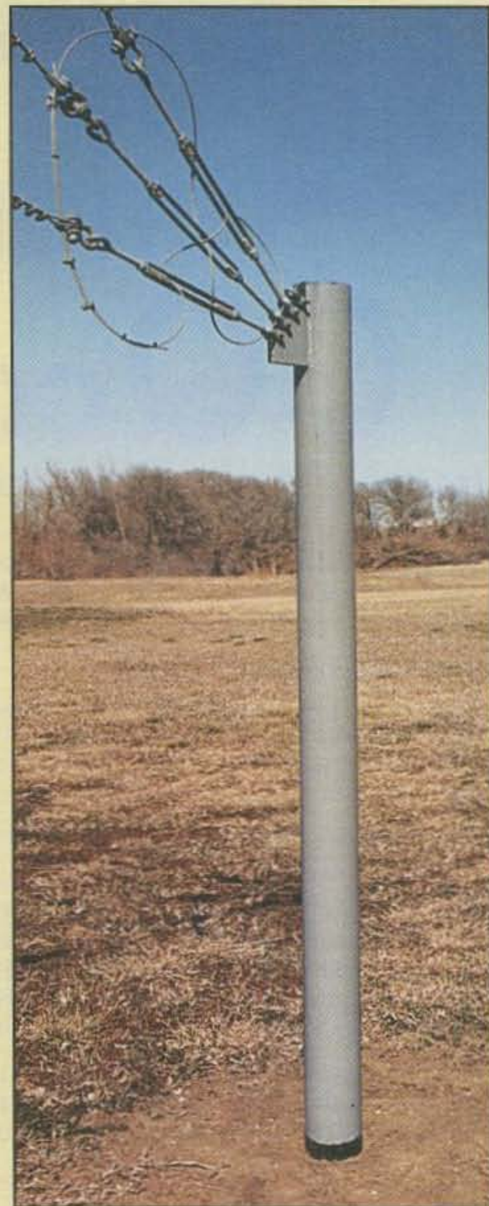
Photo A— A completed above-ground guy post with three lines attached.
