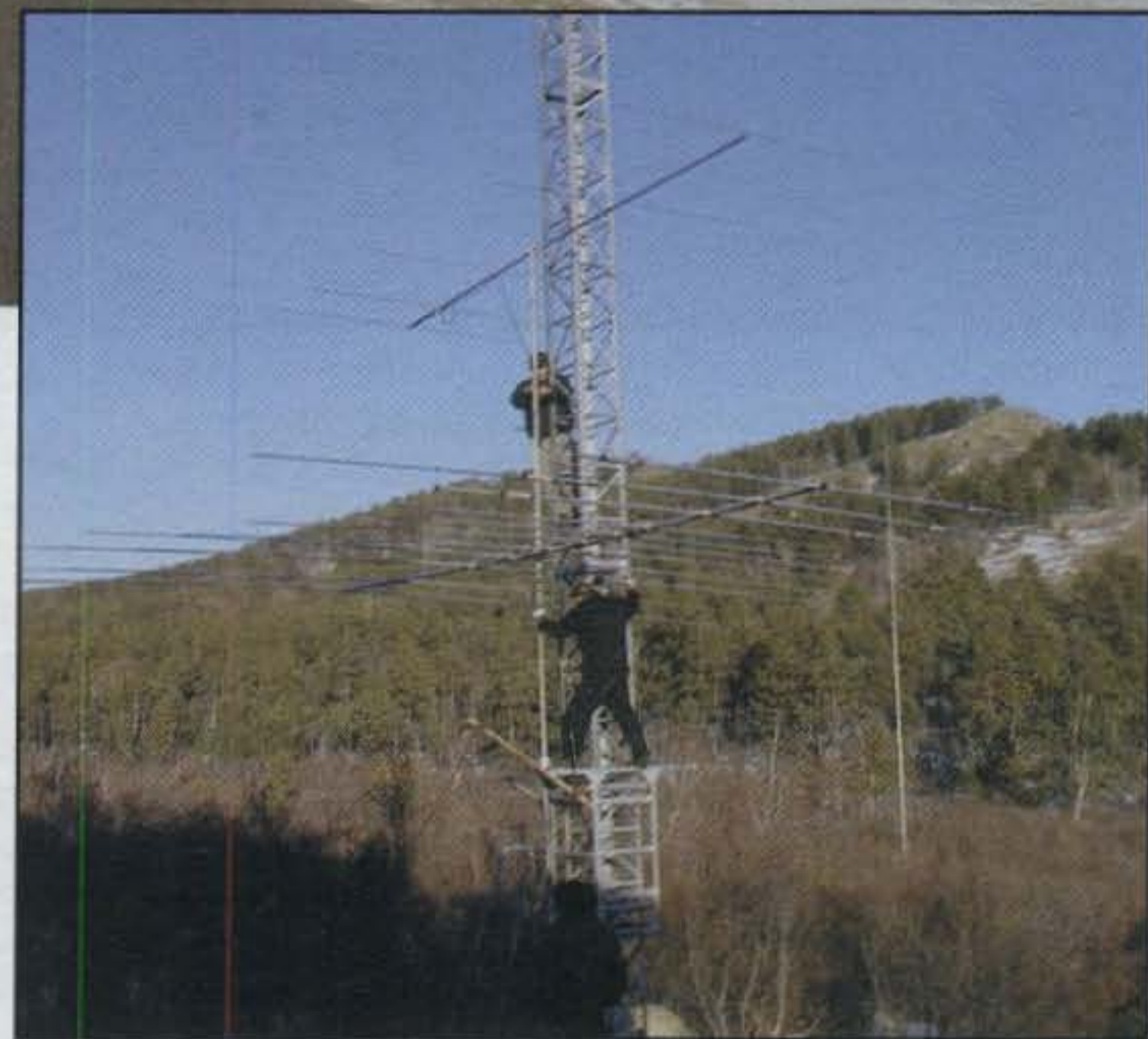
JT1BG (top) works on JT1CO's new 6 meter beam while JT1KAF (below the TH-11) holds the mast steady. (Photos by the author)
