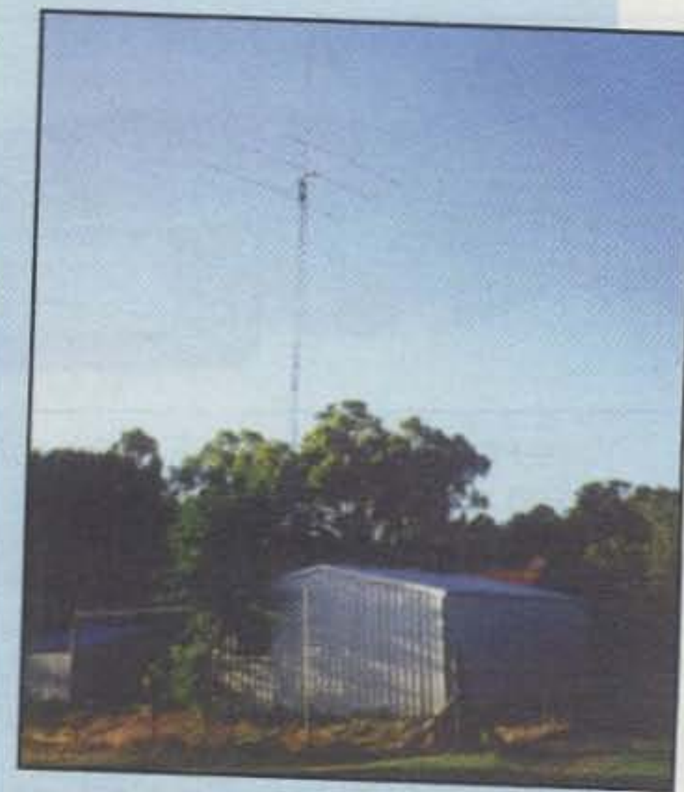
VK6VZ's 1.8 MHz inverted-Vee dipole, with its apex at 90 ft. It is supported on a fiberglass/aluminum extension pole and mounted above a rebuilt Wilson System 3 triband Yagi.
