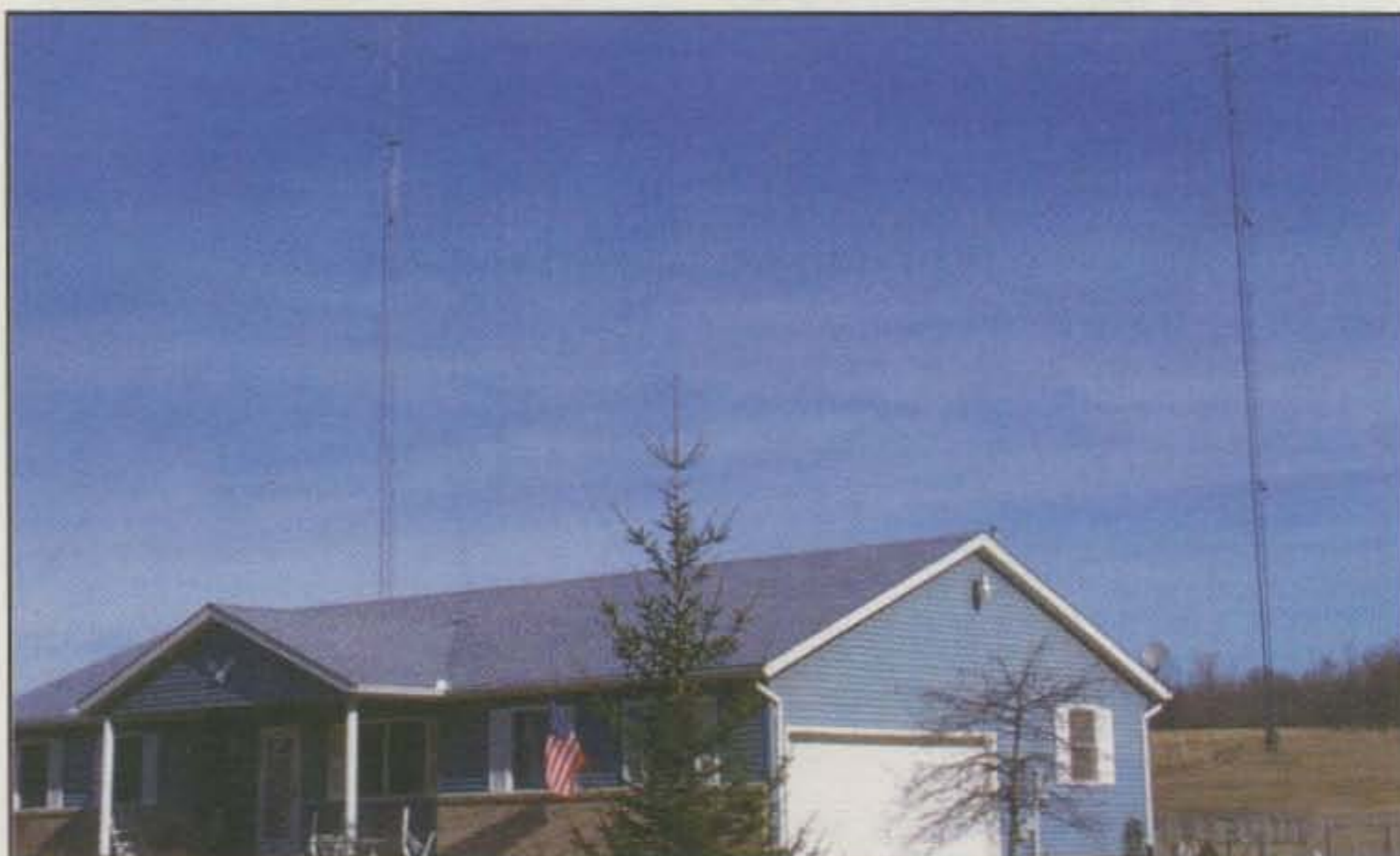
The "antenna farm" of N8BJQ. The tower on the left has monobanders for 2, 6, 10, and 15 meters. The tower on the right has a tribander stack (3) and a 2-element 40.
