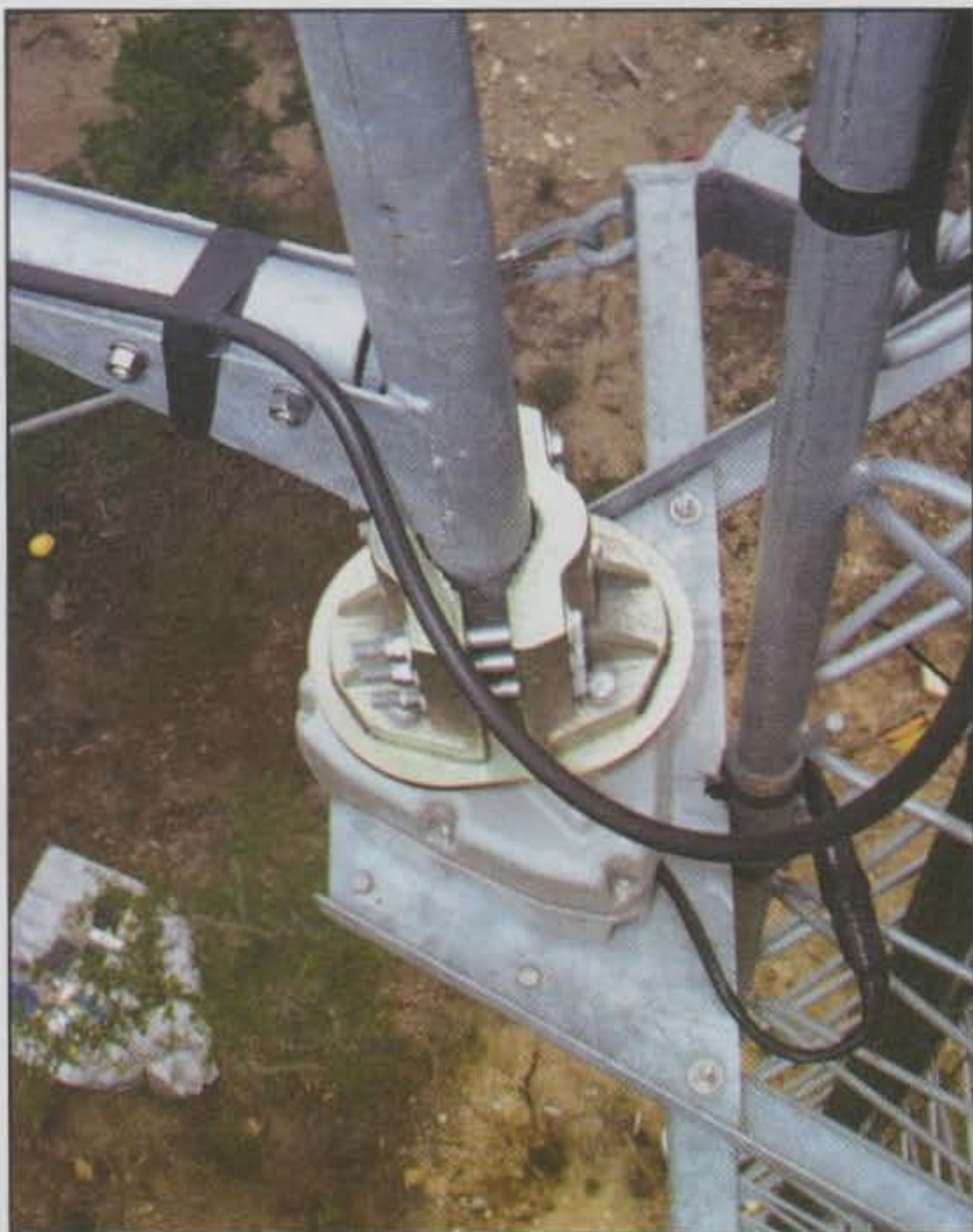
Photo C— Rotator mounting detail.
