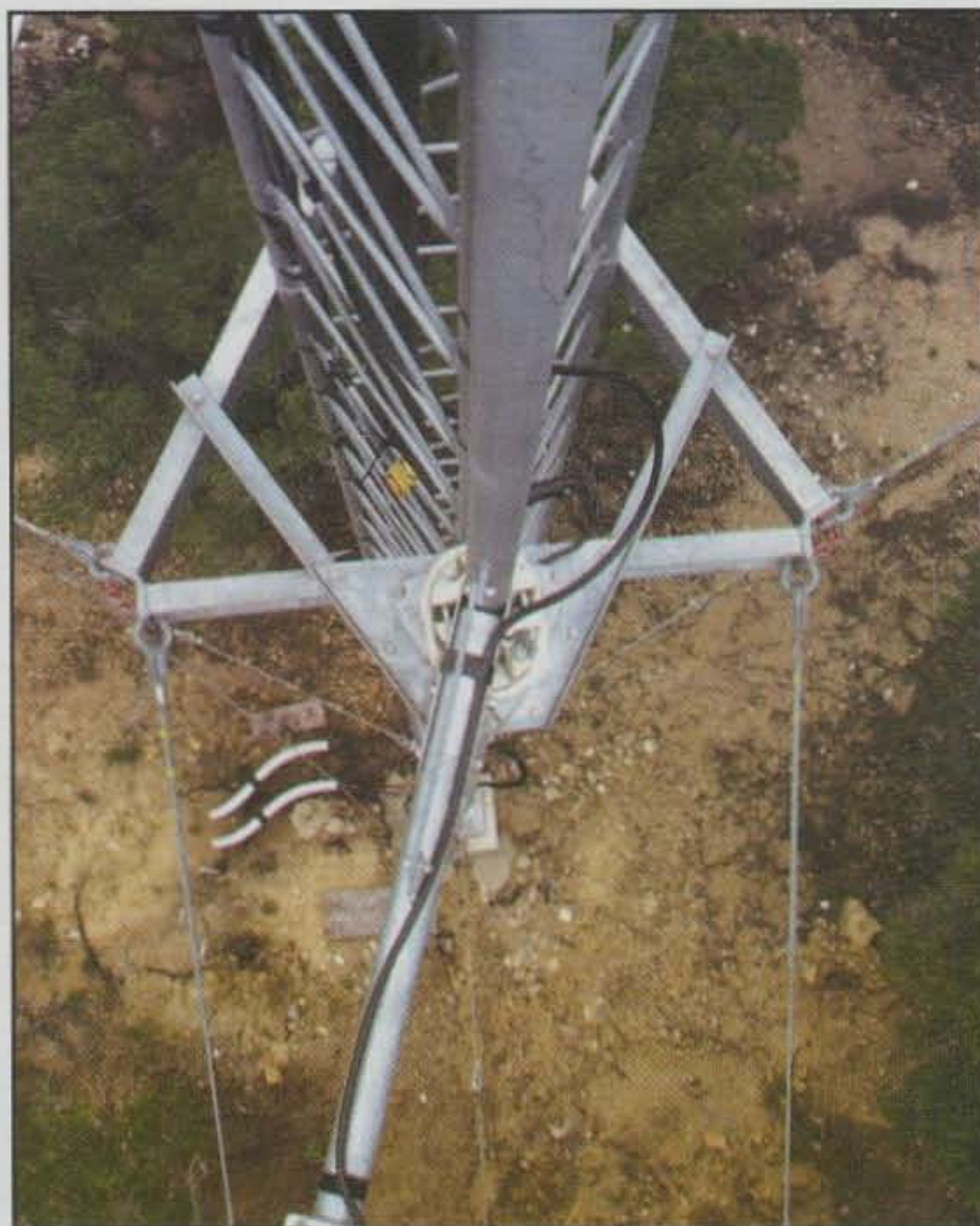
Photo D— Side-arm torque goes into guys.
