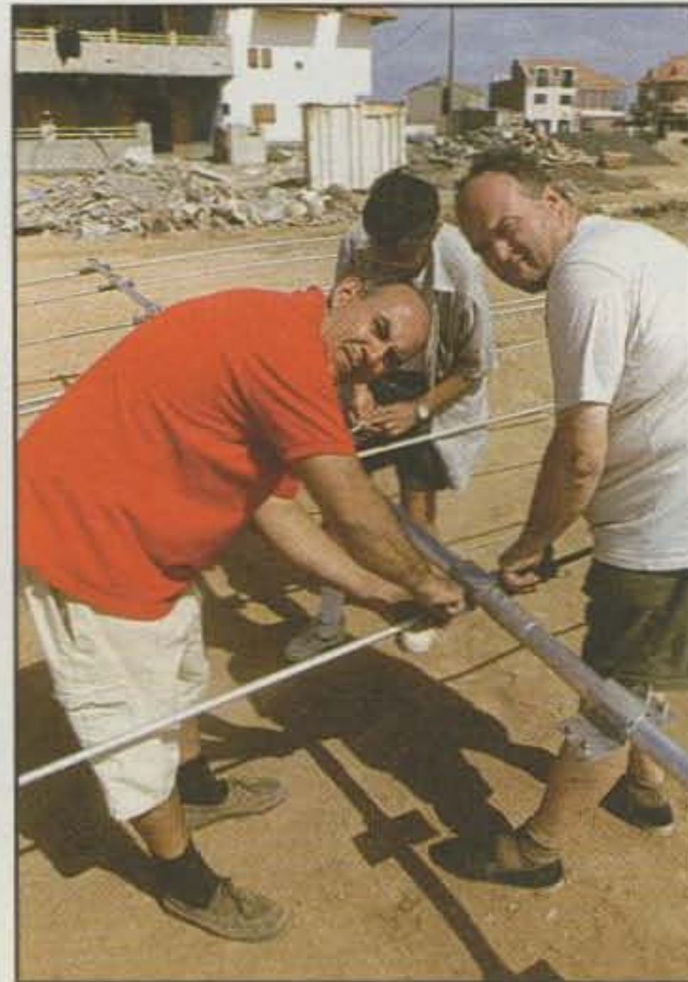
The first Force 12 array, the C19XR, grows in the hands of Santos, CT1DVV (left), Fabio, I4UFH (right), and Franco, I4LCK.
