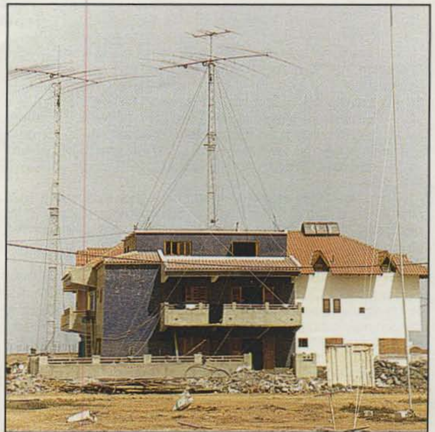
Friday and things look good! The antennas are up and ready for the contest. Now it's time to work on the radios!
