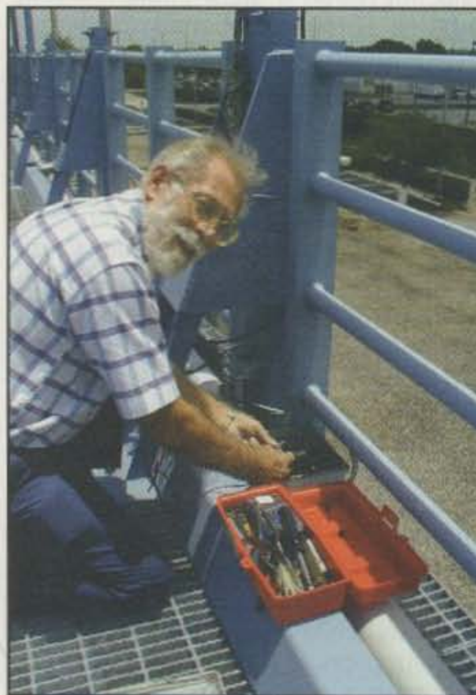
John McHugh, KU4GY, checks all the lightning arrestors and connectors while Nick Pikarsky, N4EVB, makes antenna adjustments. (WD4JR photos)
