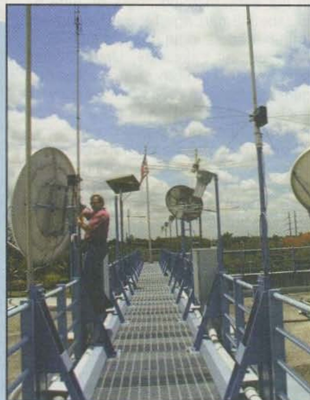
John McHugh, KU4GY, checks all the lightning arrestors and connectors while Nick Pikarsky, N4EVB, makes antenna adjustments. (WD4JR photos)
