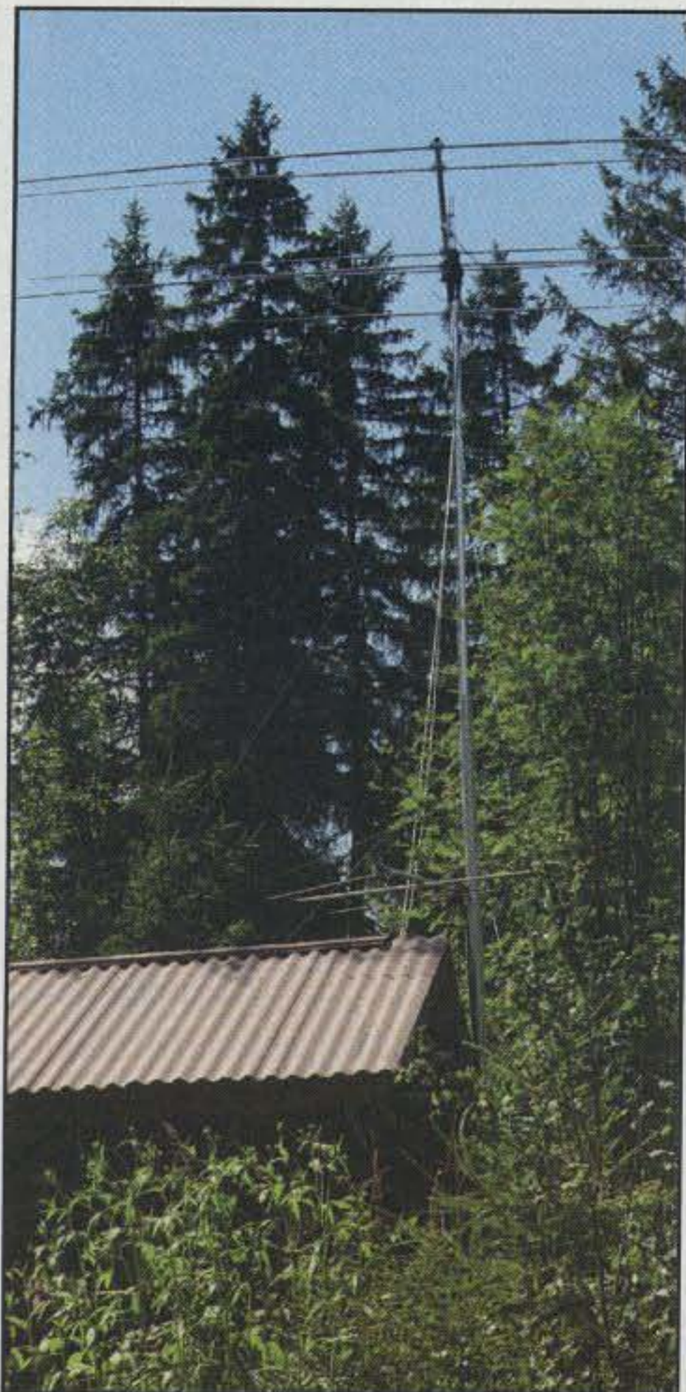
There were 52 identical antenna installations like this for each WRTC 2002 team.
