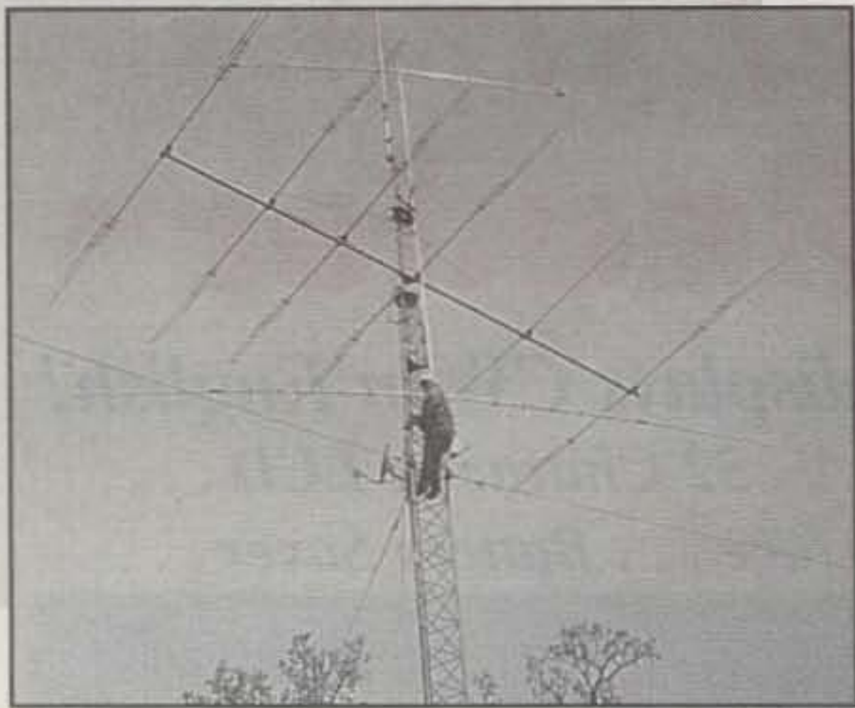
Photo C— WRØU removing antenna elements.
