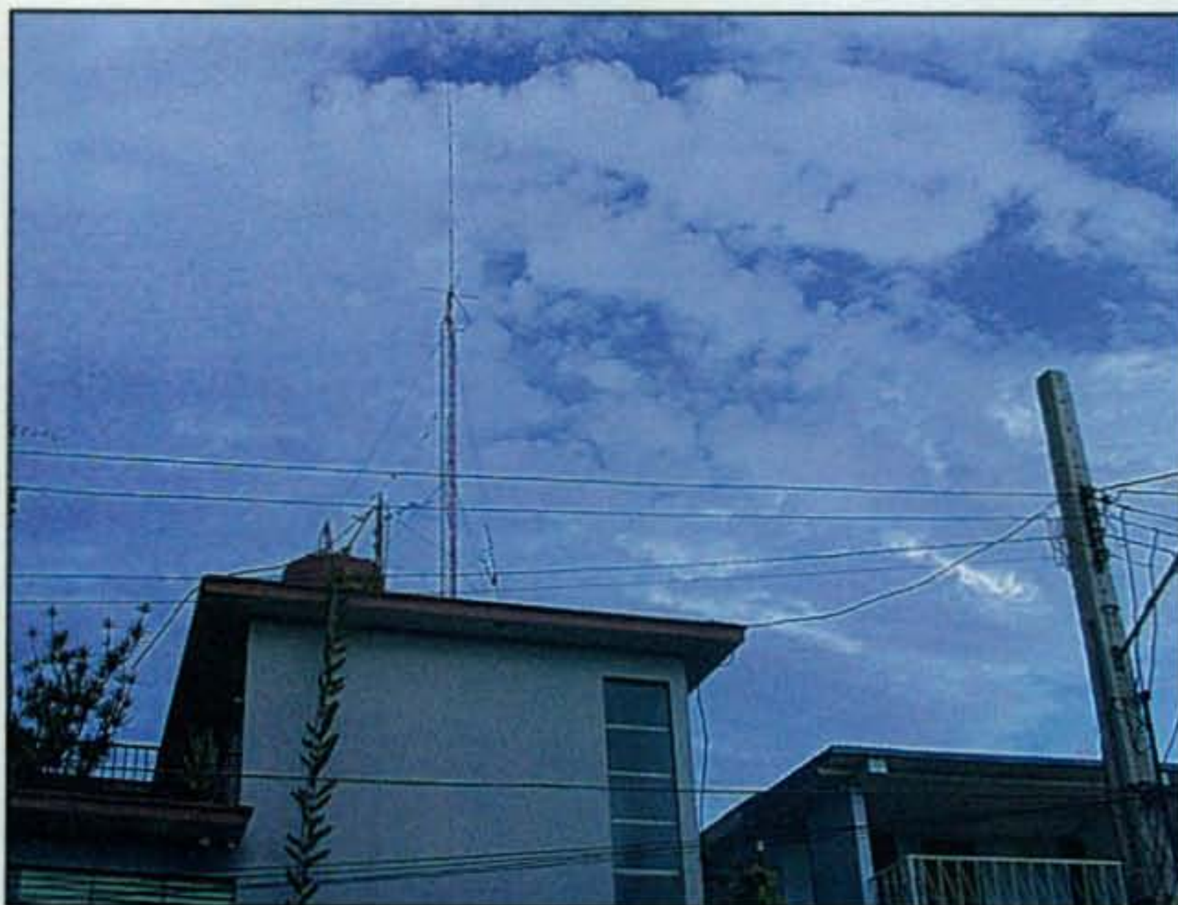
Photo A— Full-size, 2 meter, omnidirectional, vertically polarized antenna at CO2KK's QTH using three 5/8 -wavelengths elements. With its estimated 6 dB gain over a dipole, it's my standard of comparison for 2 meter FM work.
