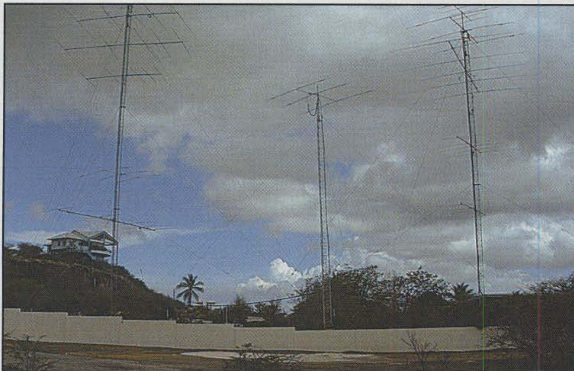
Nothing like a few beams to keep the rate up at PJ2T! (Photo via K8NZ)
