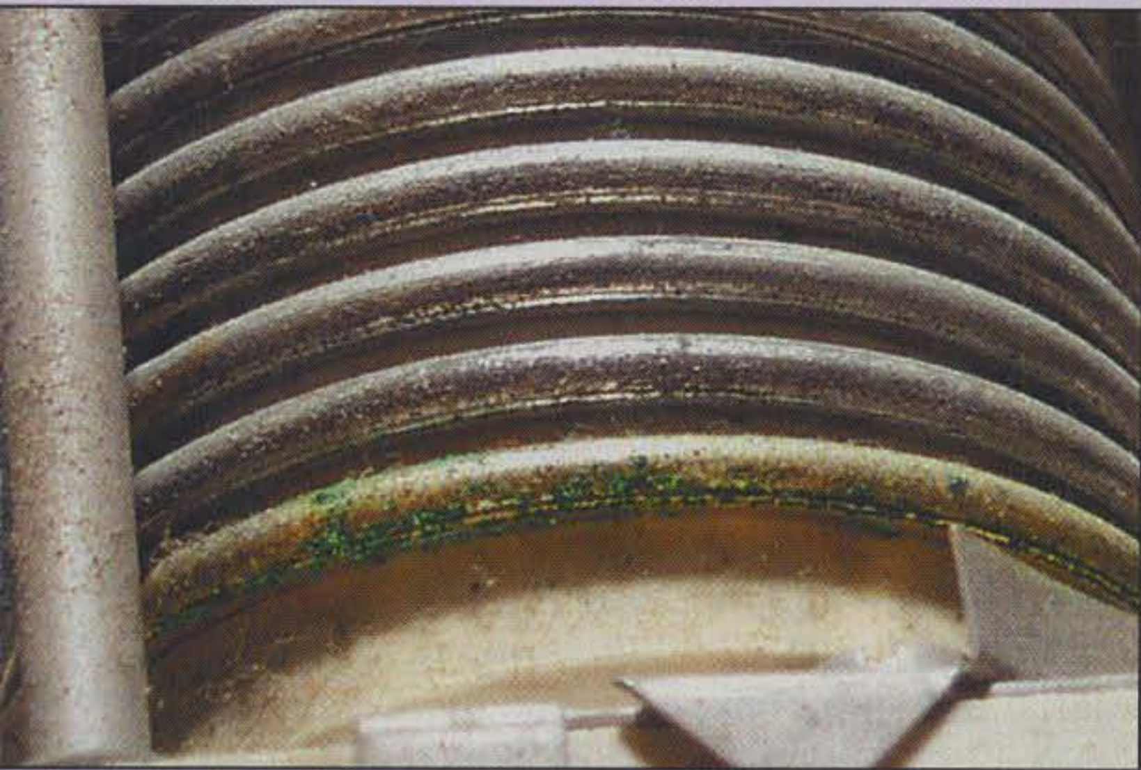
Green oxidation inside a linear amplifier, caused by bacteria.
