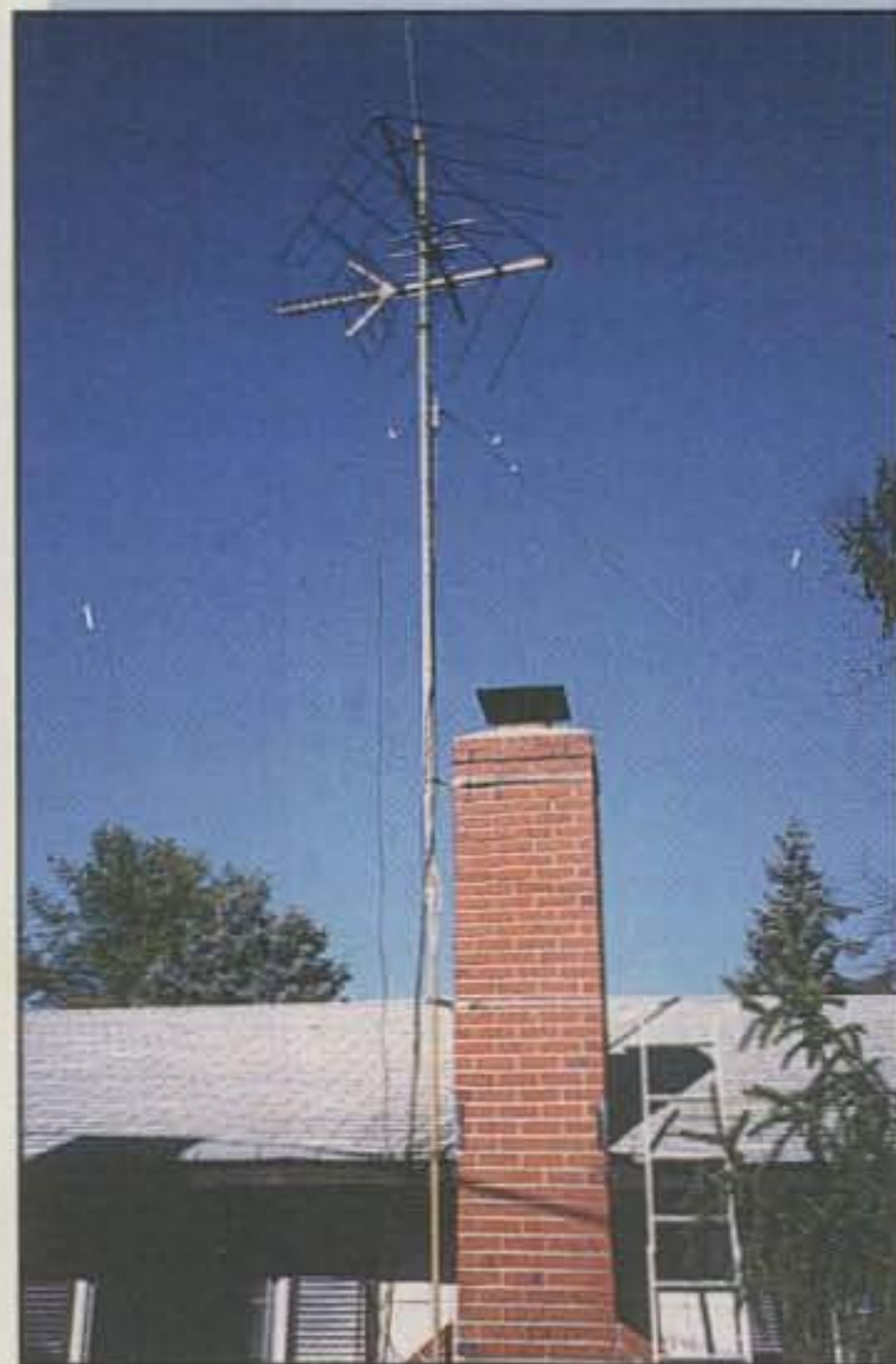
Photo B- Sharing space on a metal mast attached to the chimney made it essential to use a coax feedline instead of open-wire line, which might have been more tolerant of mismatches. However, ladder line could interact with the metal mast, causing it to radiate.
