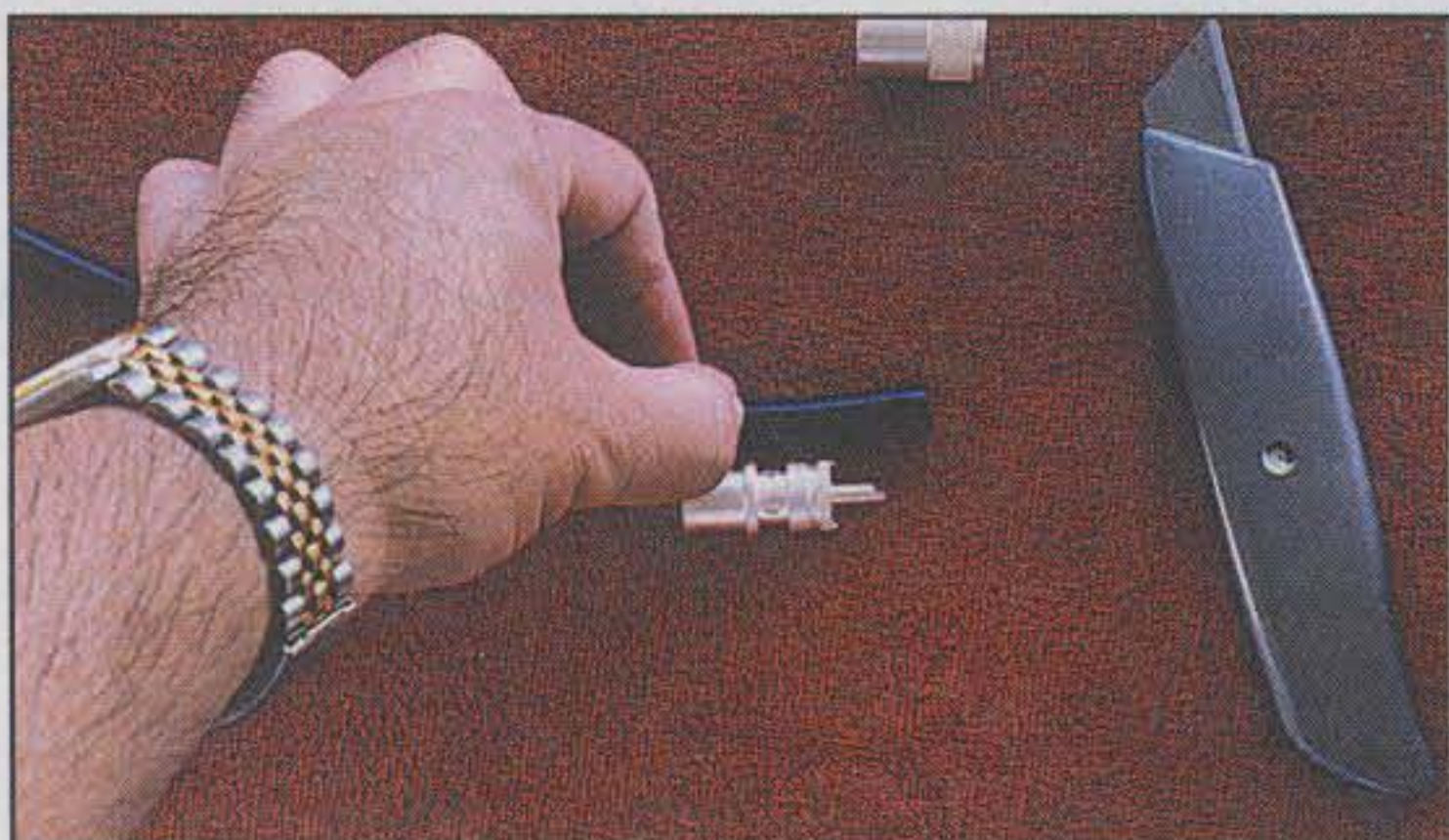
Photo 3— No need to measure. My thumb indicates where the outer jacket needs to be removed. Notice that the length of cable is slightly longer than the connector length, as indicated by the center pin.
