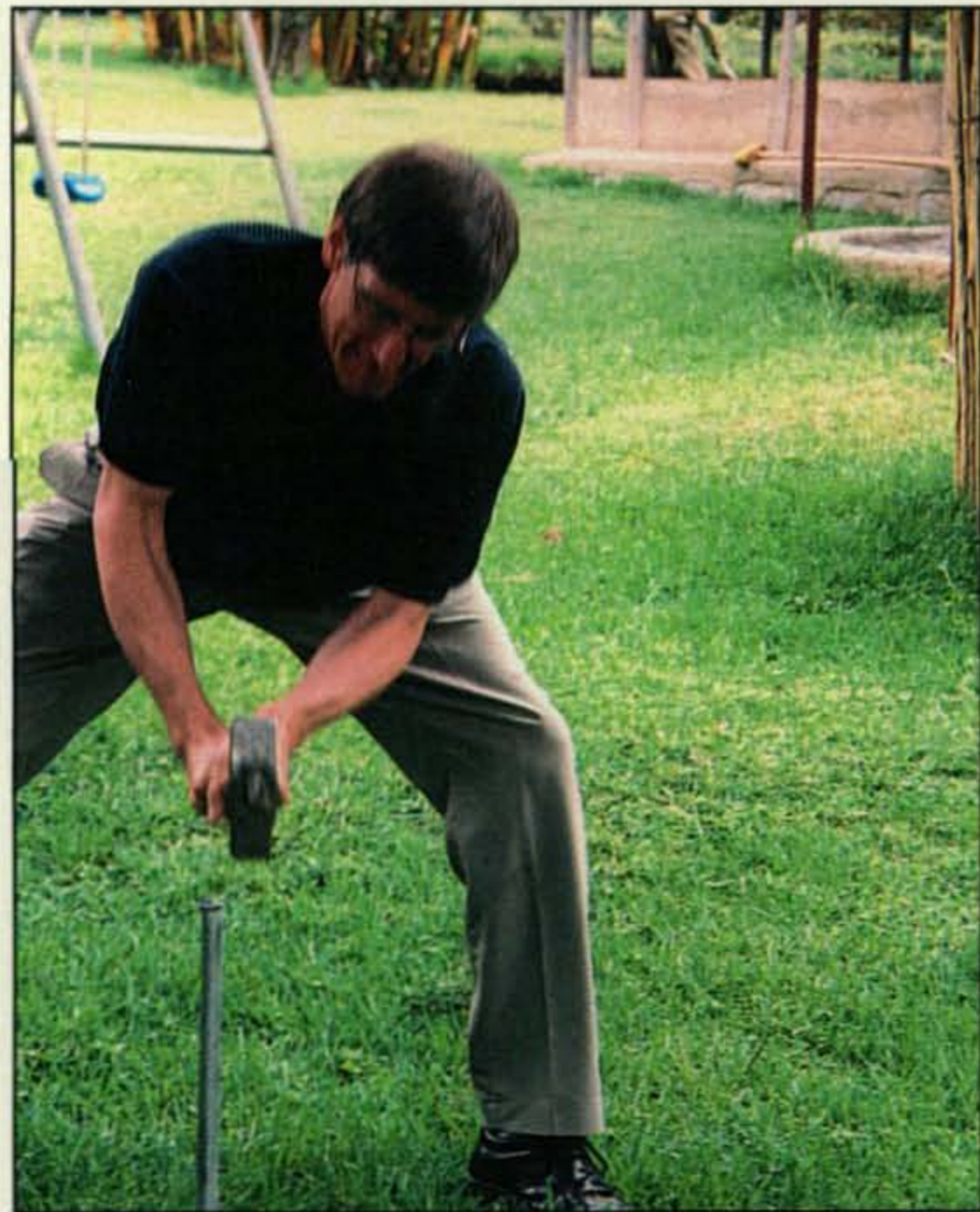
Dale, N3BNA, hard at work pounding in a ground rod for the K9AY receiving antenna he brought to Ethiopia in his "care package" for Paul, along with an amplifier and a variety of other gear.
