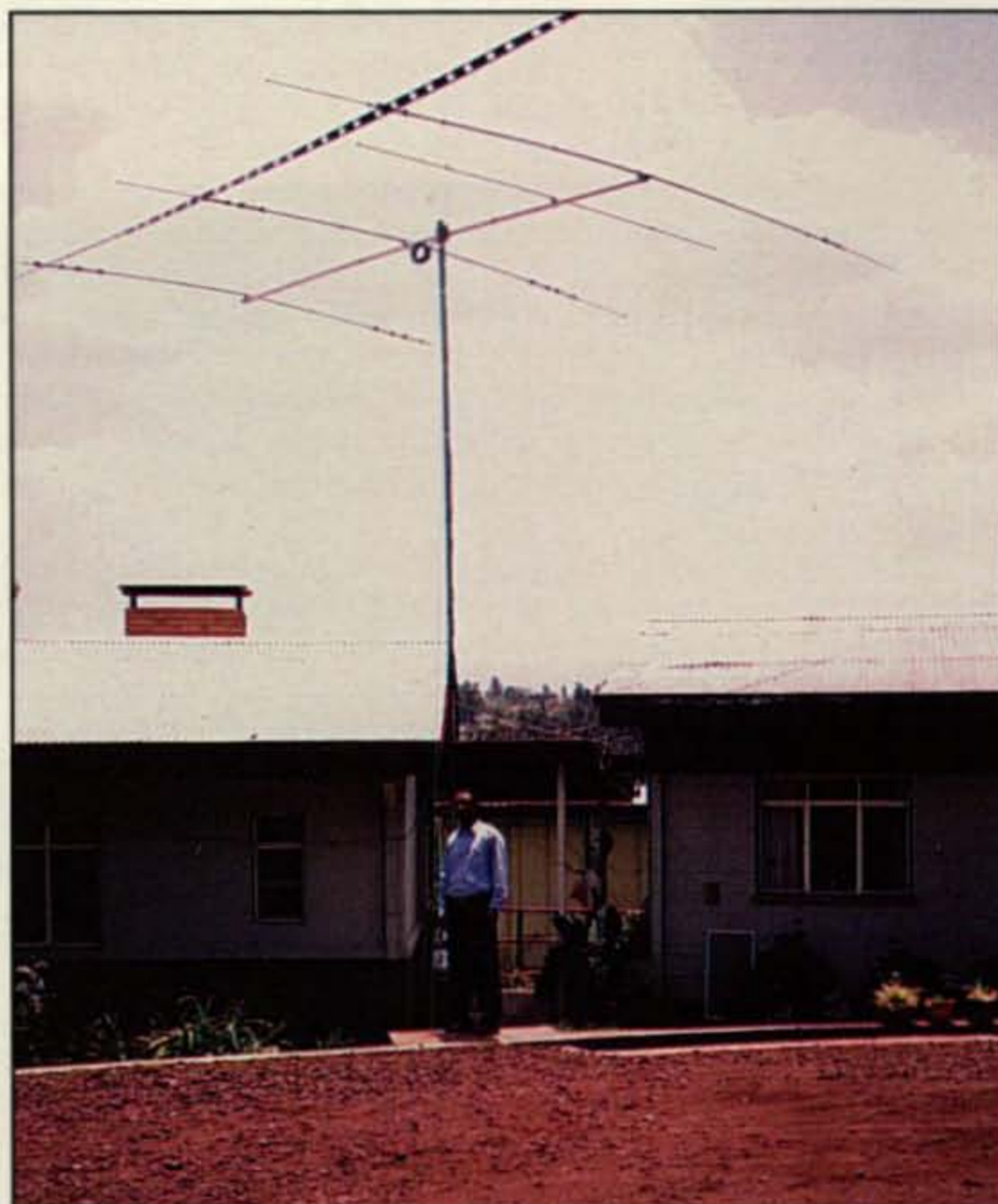
Higher frequency bands at ET3PMW were initially handled with this used Cushcraft A3 mounted at 30 feet. The feed line for the 160 meter antenna is visible in the foreground. The person in the photo is Yohannes, who helped Paul with his antenna projects.
