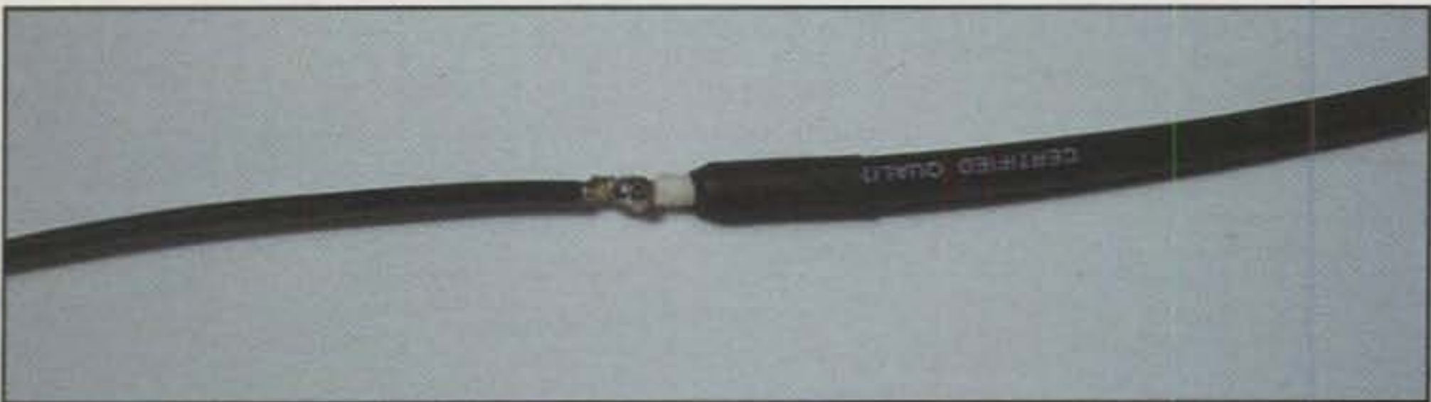
Photo B— Connection of inner end of coax section (closer to center). Note that only the center conductor is connected to the wire.
