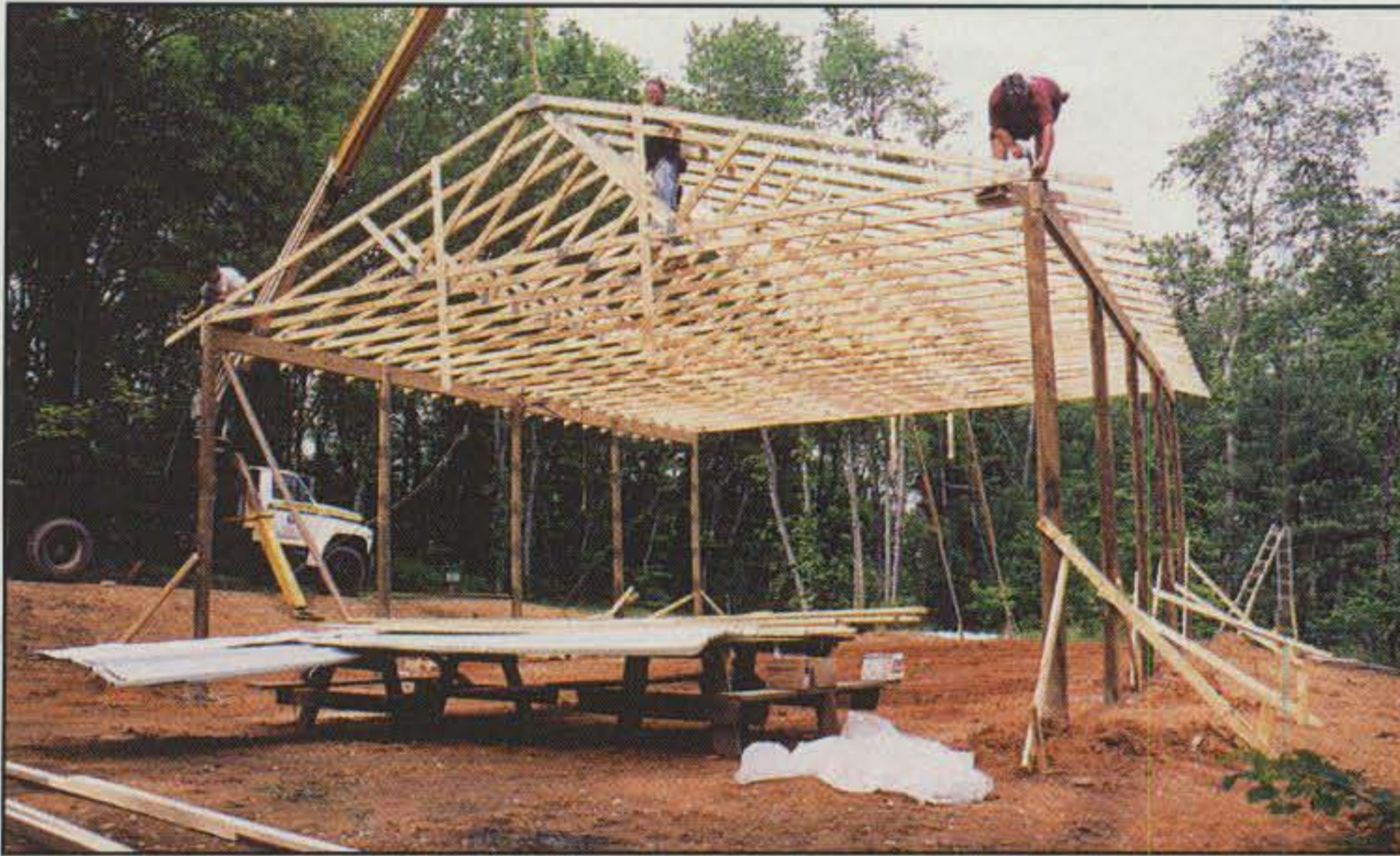
The 30' x 40' Goforth Ham Shack shelter during construction.
