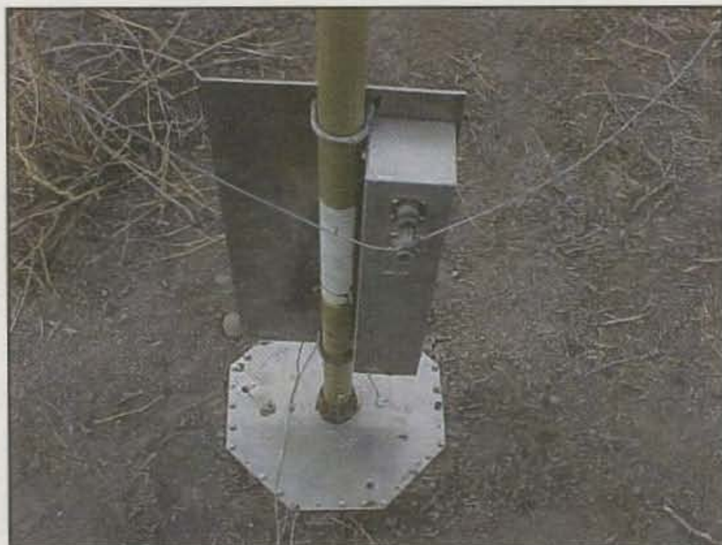
Photo C— Base of the antenna. The box holds the tuning capacitor and the plate to which it is mounted attaches the capacitor unit to the antenna.
