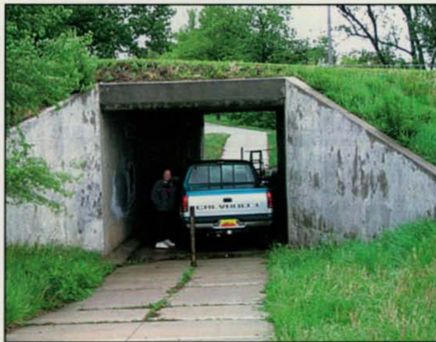
Somehow Matt, KØTEA, and Tom, WBØYWN, got their truck safely inside this pedestrian underpass on a rainy Nebraska morning. (Photo courtesy of KØTEA)
