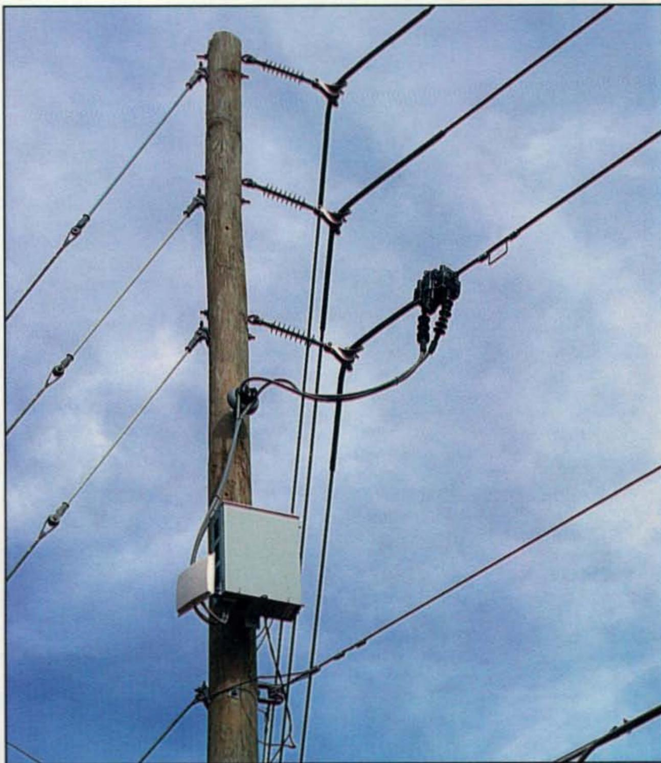
The box on this power pole is called an "injector" and it injects the BPL signals onto the overhead power line. The small white box on the left of the bigger gray box is a Wi-Fi antenna, which receives data from a substation a few blocks away. It is then inductively coupled to one phase of the power line with the two big clamps seen on the wire. (Photos by the author)
