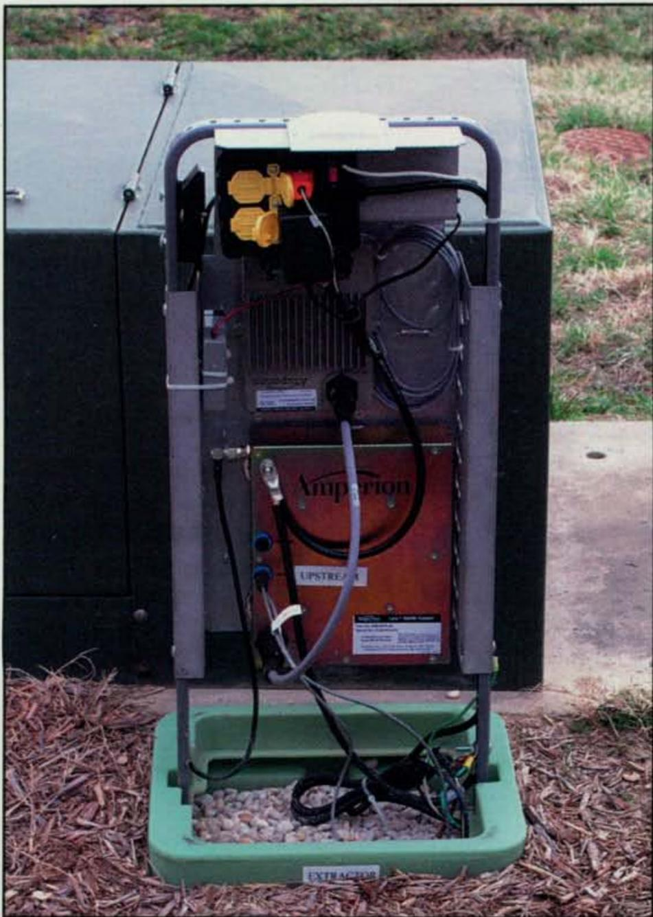
Inside the BPL "extractor," the broadband signals are taken off the power line and fed to a "Wi-Fi" antenna for final transmission into subscribers' homes. Amperion uses Wi-Fi for this last leg; other companies take the signal all the way into each house on the power line.
