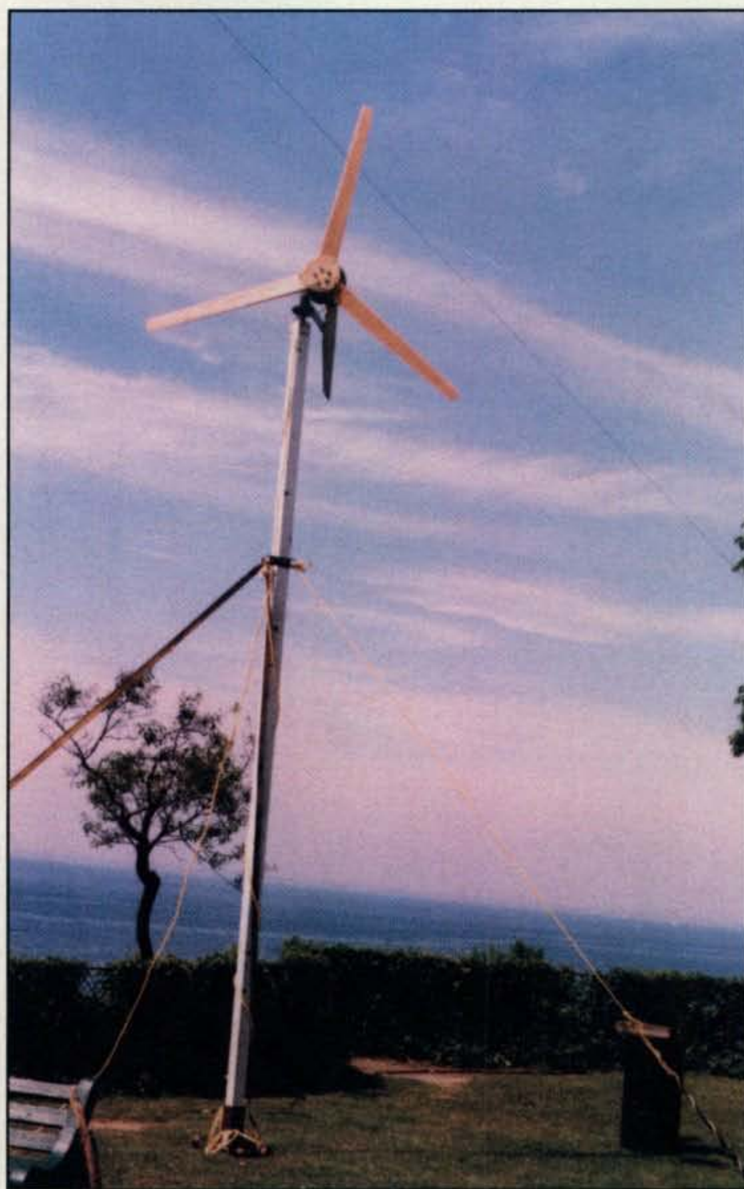
Photo C— The final installation of Roy's windmill at the Peconic ARC Field Day site, with Long Island Sound in the background. At times the wind speed was quite high. (Photo by Ken, WB2AMU)
