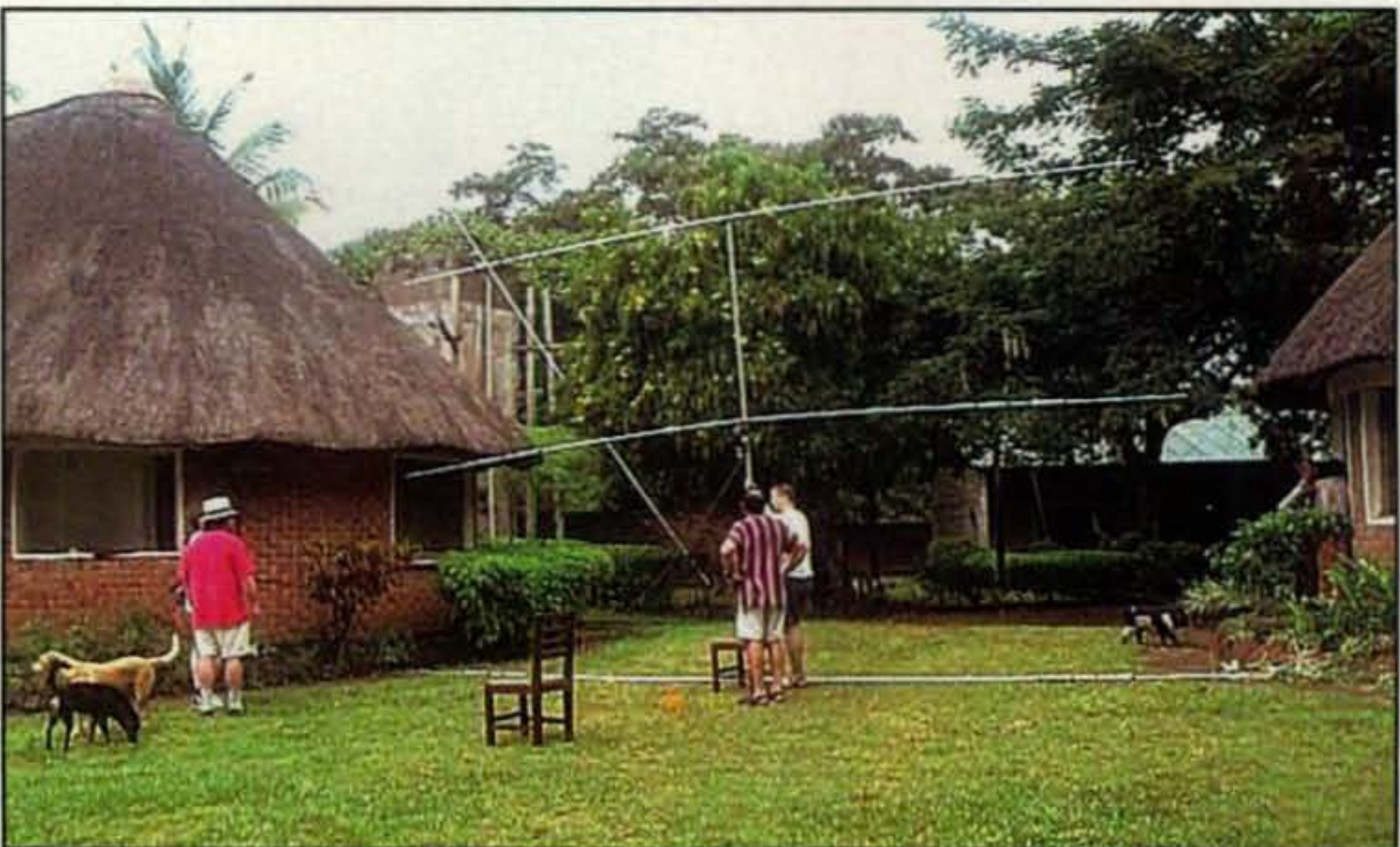
Assembling the 10-metre Yagi. In the background (behind the building) is the water tower, which became the support for the Cushcraft A3S.
