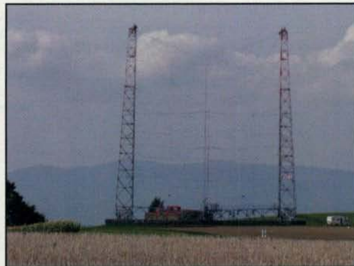
The antenna system used by the broadcast station of Radio Switzerland International.
