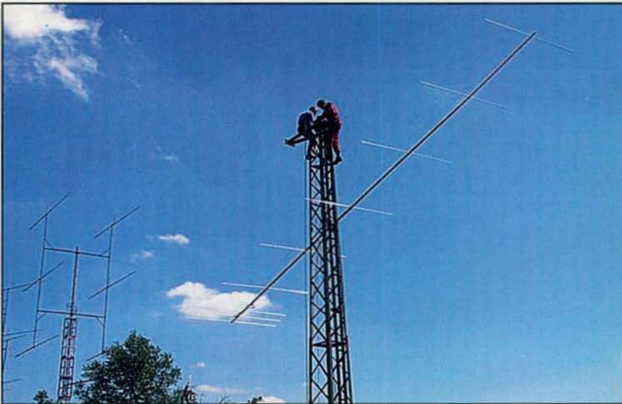
OK1HGN and OK1RI of Radioklub OK1KIM putting up the 6-meter Yagi just a few hours before the contest. Note the double H-frame 2-meter hardware in the background.
