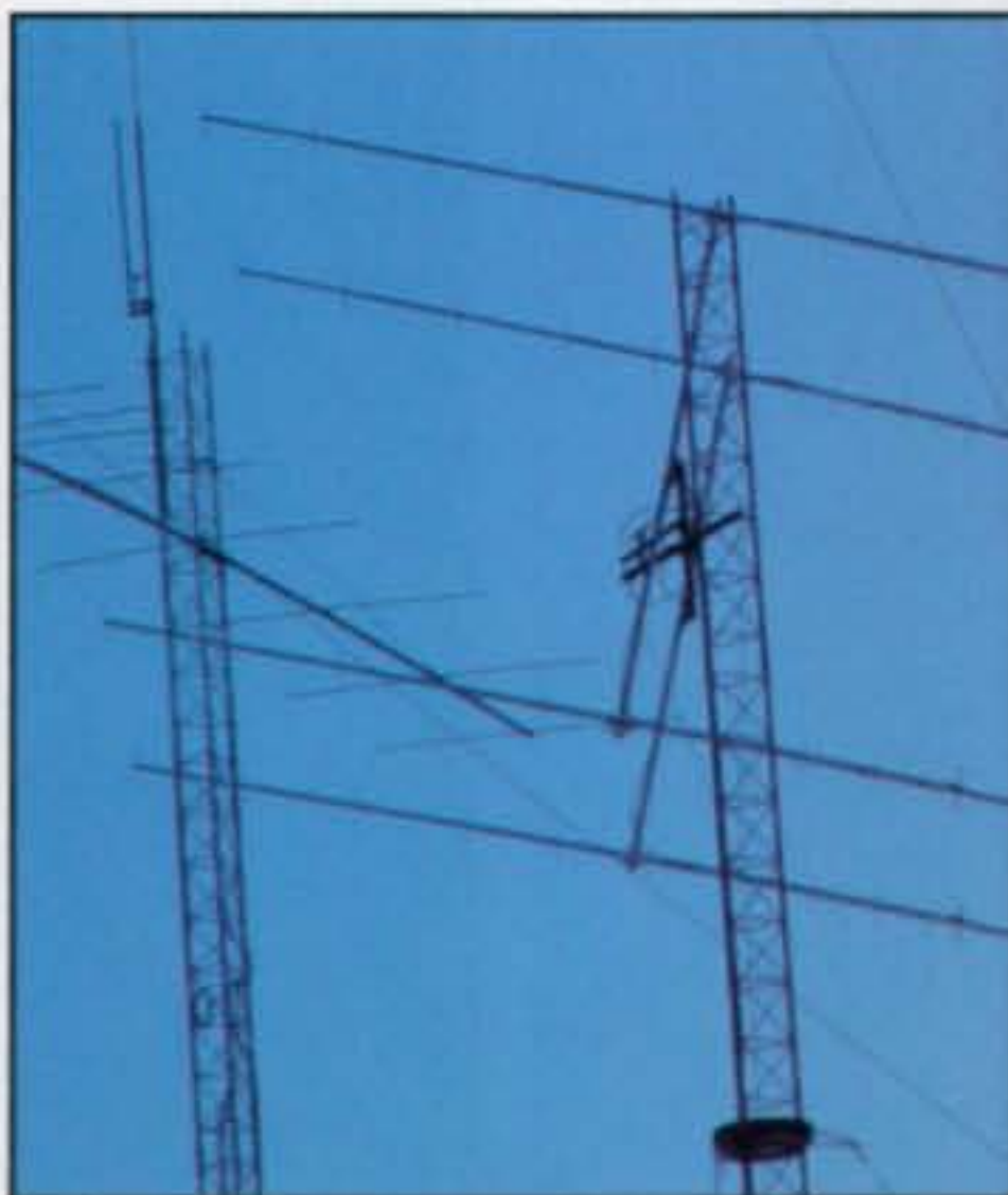
The 2-meter EME array atop the rotating tower. To the left side is a partial view of one of the two 8-element, 42-foot boom, 6-meter stacked Yagis mounted on a separate rotating tower.
