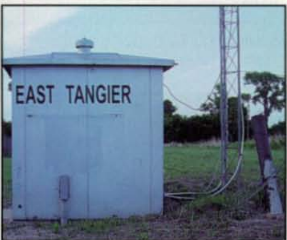
This building came from the Santa Fe Railroad. It houses a 70-cm repeater and will house the tuning units for the HF vertical.
