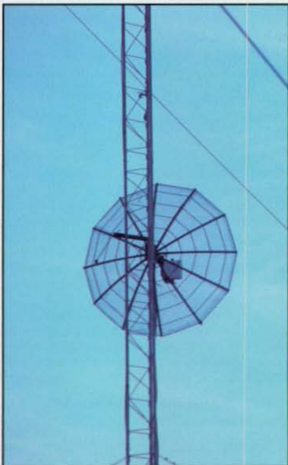
Dish antenna used for WiFi.
