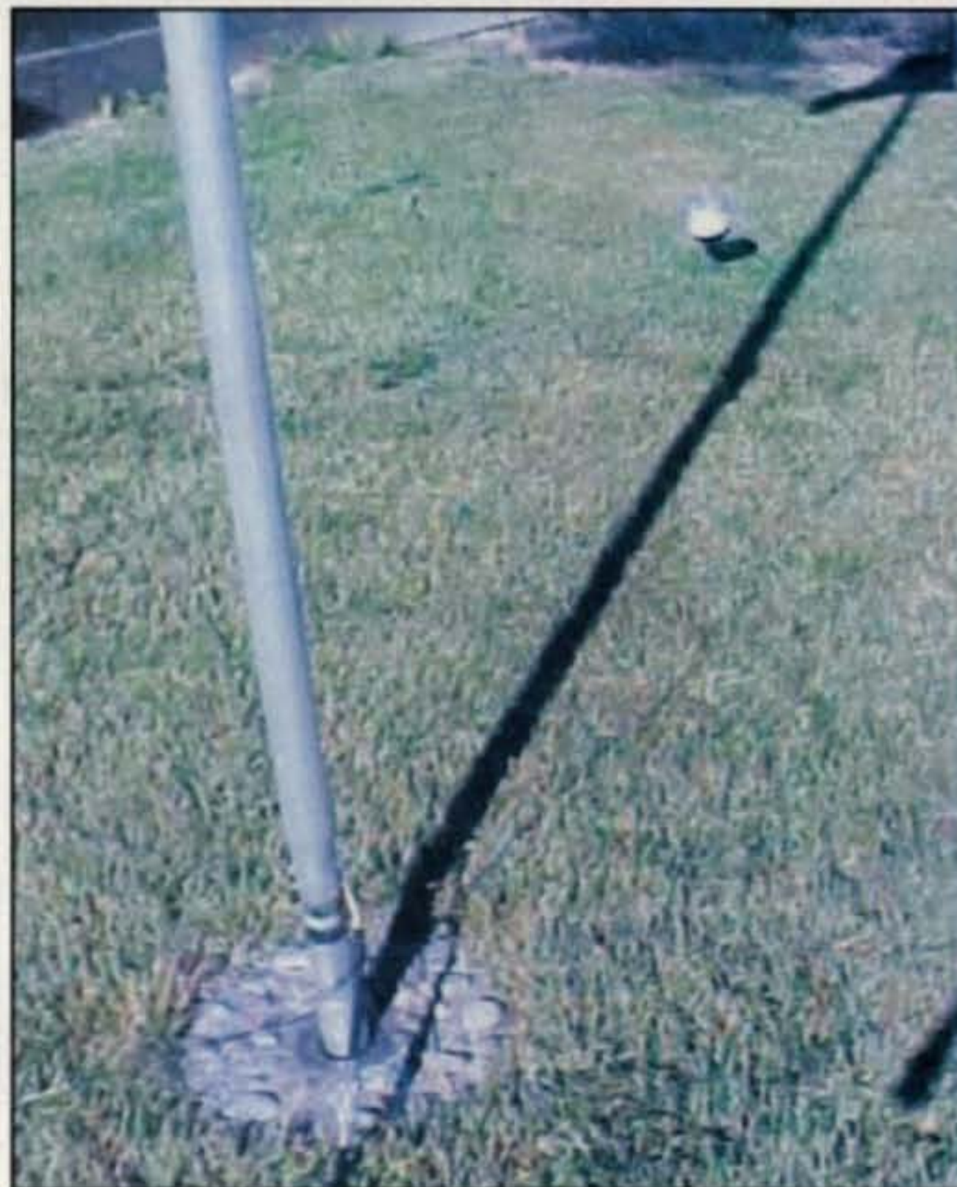
Photo 2— This view shows how the Force 12 antenna fits onto its short base, which you fit into quick-setting cement. Look carefully and you can see one radial wire disappearing into the grass.
