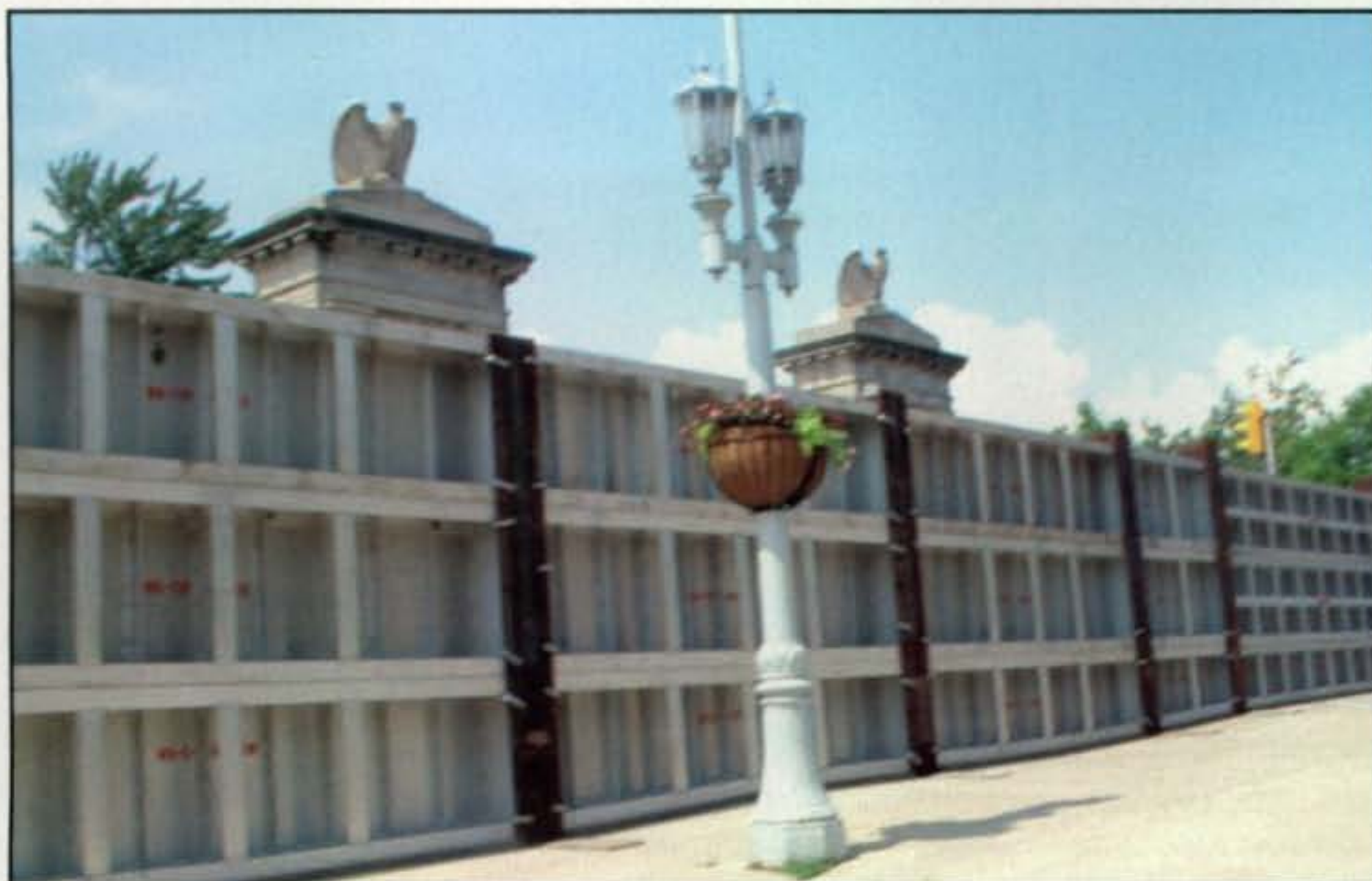
Flood gates across bridges and other protective measures along the Susquehanna River minimized serious damage in the Wilkes Barre area, where more than 100,000 people were evacuated. (Photo courtesy of KB3MLD)
