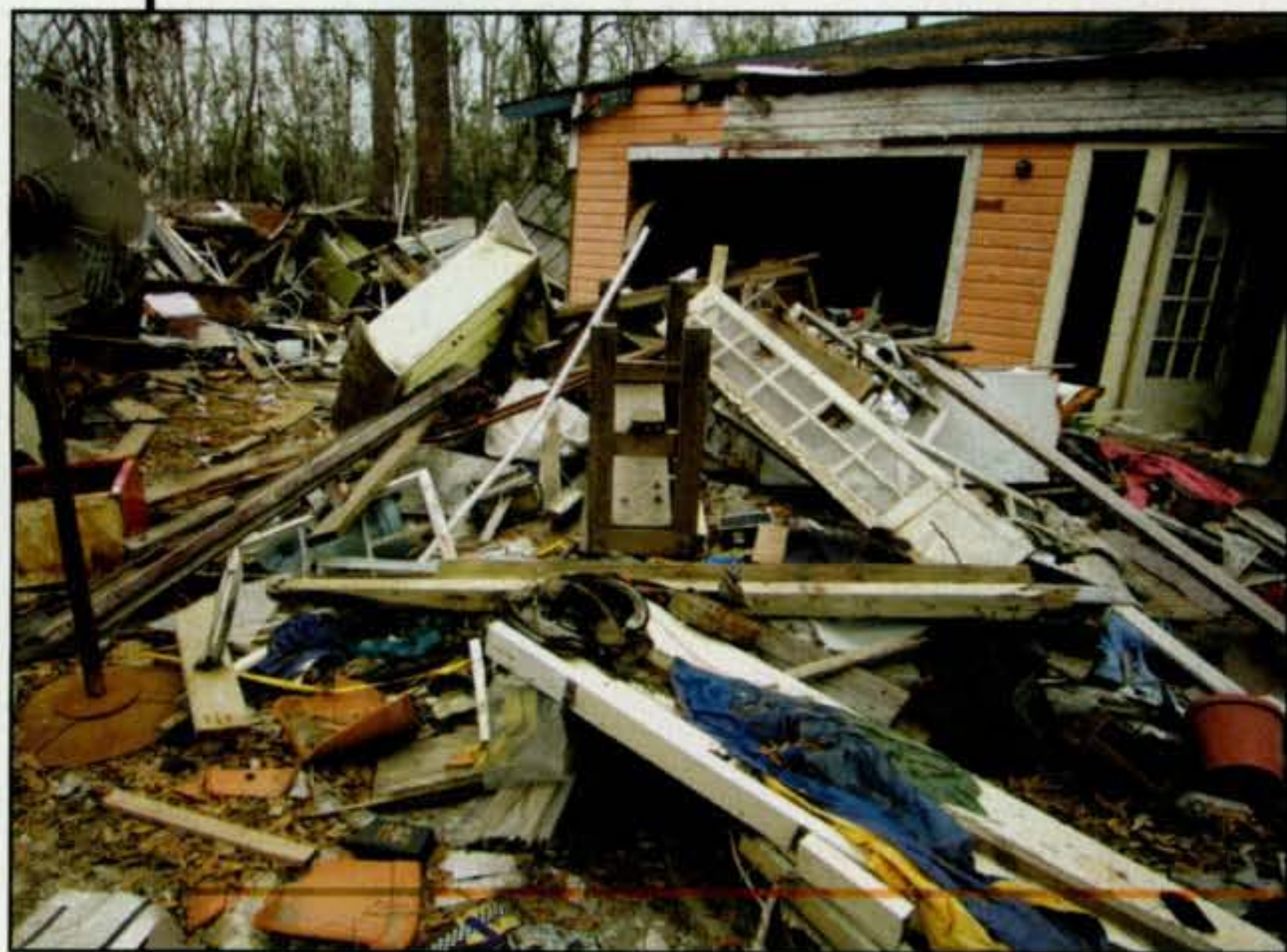
The destruction of this home is a result of Hurricane Katrina's landfall in a small Mississippi coastal town. Nearly 92,000 people lost their lives to disasters in 2005. (Photo courtesy of Leif Skoogfors/FEMA photo)
