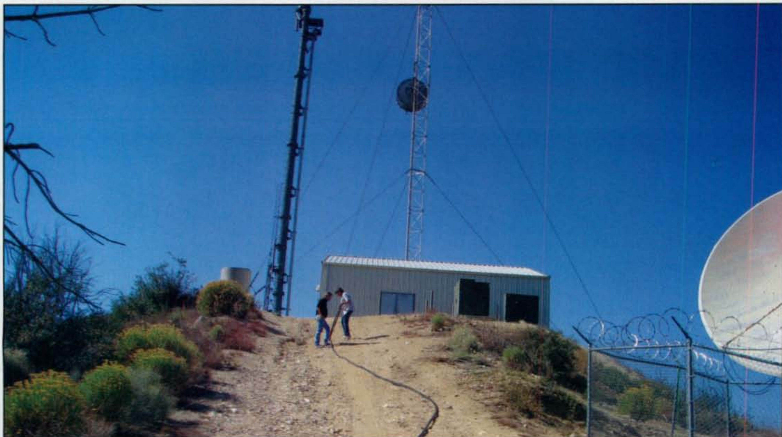
Photo C— Repeaters are often installed in remote locations. This 900-MHz system is on a mountain ridge at more than 2000 feet elevation. (Photo by Glenn Allen, KE6HPZ)
