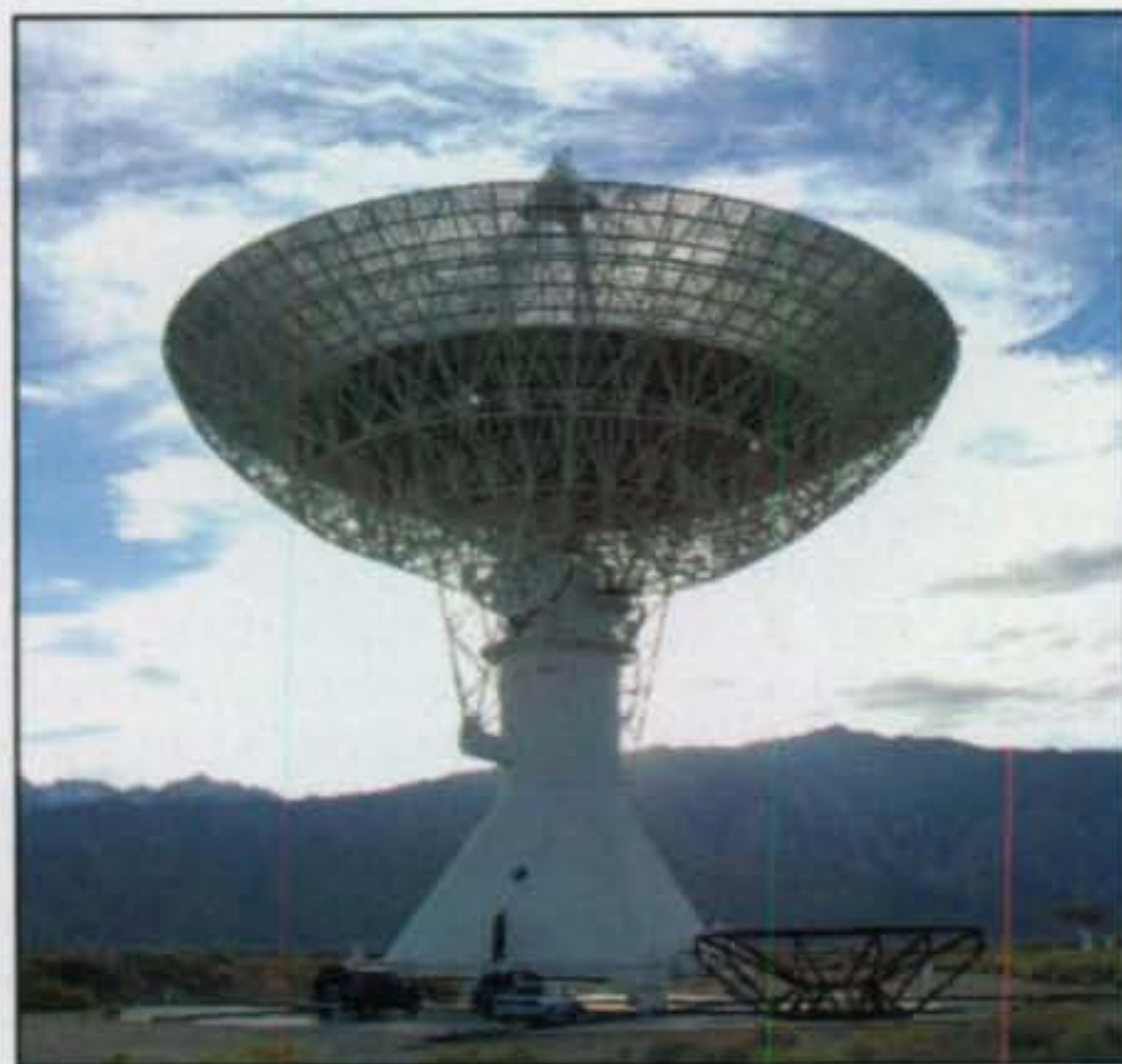
Photo A— The Owens Valley Radio Observatory (OVRO) 40-meter diameter dish antenna is actually a radio telescope that is being used to transmit 1296-MHz and 10368-MHz ham radio signals to the Moon and back to Earth. This is a fairly extreme example of equipment needed to move VHF and above signals beyond line of sight. (Photo by Rich Whited, KG6JKJ)
