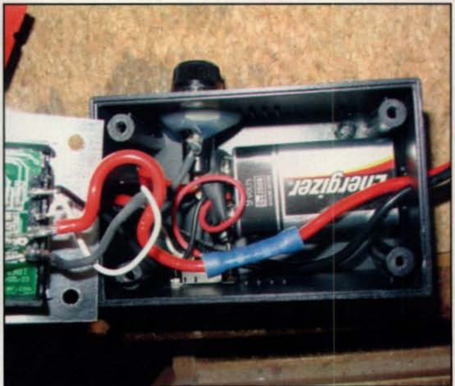
Photo D— Internal wiring view.
