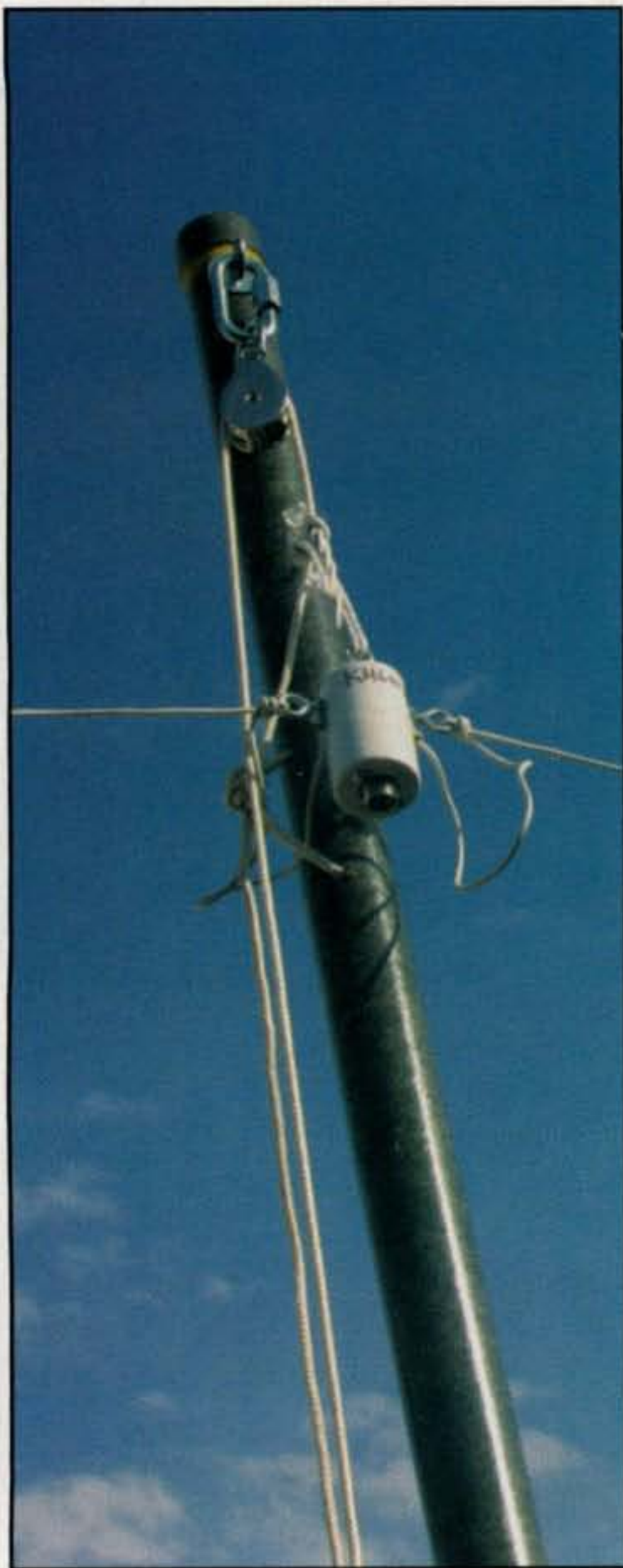
Photo 8— The completed antenna is raised to the top of the mast by pulling on the support line. When you do this, make sure the coax feedline is attached to the center insulator. . . .
