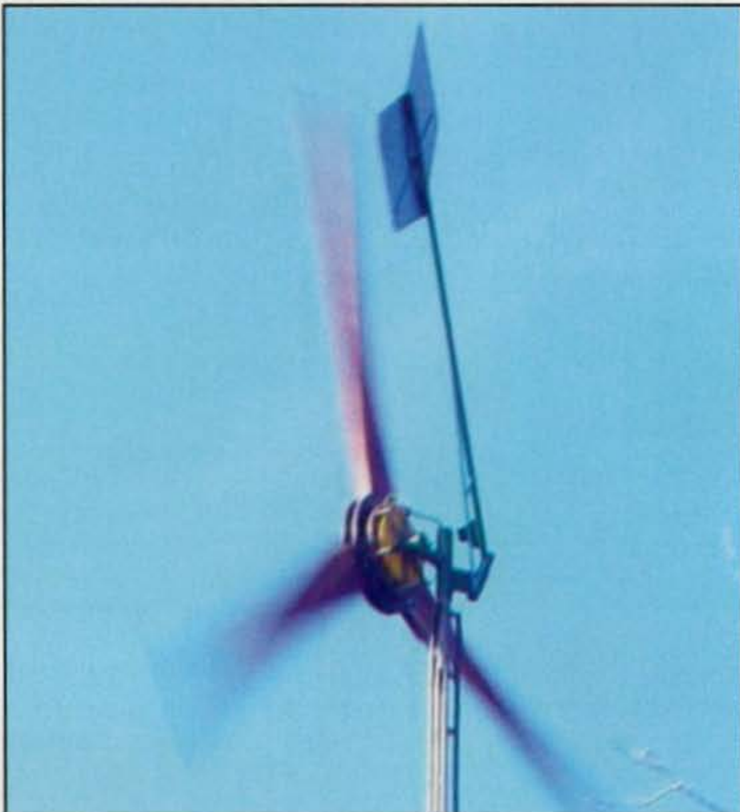
Photo D— In the presence of high winds (over 10 or 15 mph) the wind turbine furls for self-protection, and continues developing maximum output. (Photo courtesy of Dan Bartmann, KC0VSV)
