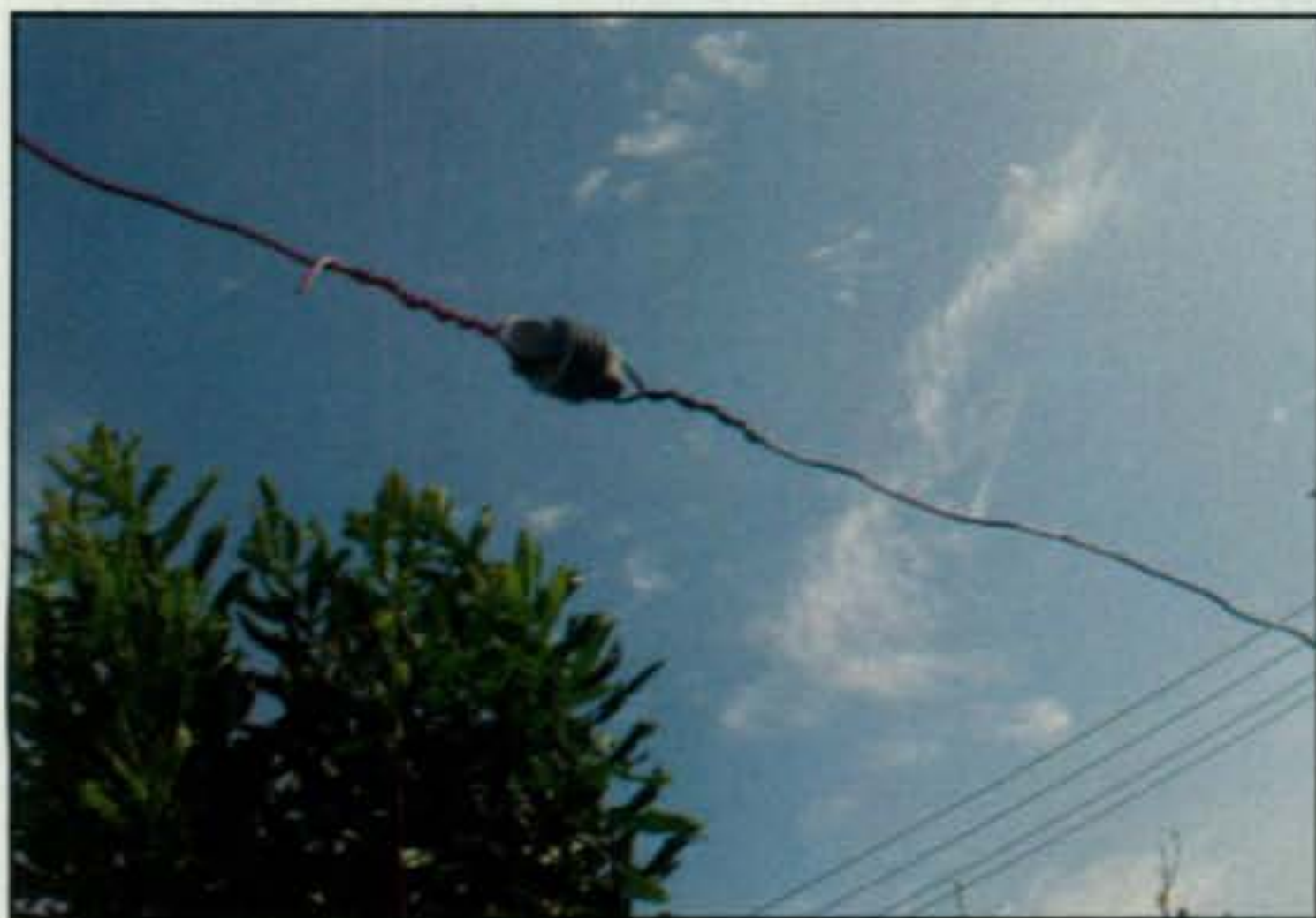
Photo 5— If using solid wire, the ends can be wrapped back upon themselves as shown. This photo also illustrates what the far end of a wire antenna and its insulator looks like.
