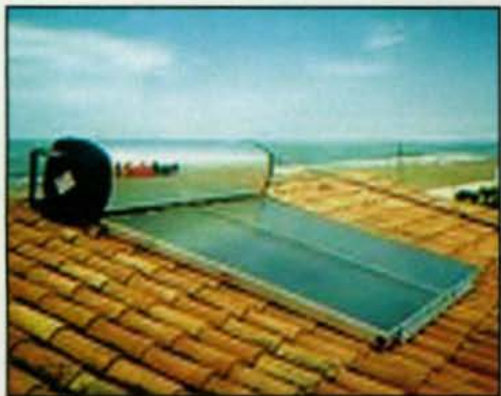
Photo E— One of the top energy guzzlers in a typical home is an electric water heater. Replacing it with a solar water heater similar to this Solahart unit reduces one's electrical needs quite noticeably. Details on the heater can be found at < www.solahart.com >.
