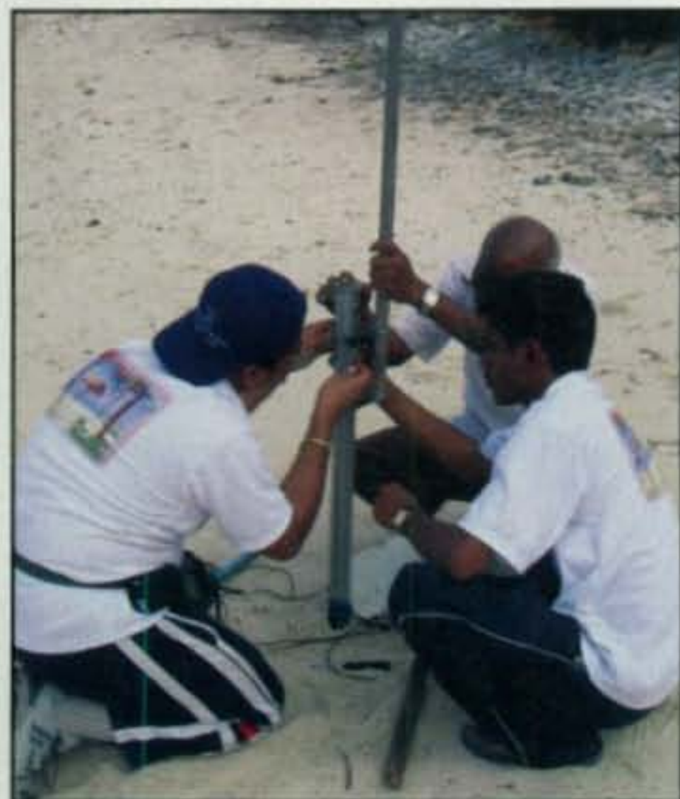
A three-band Fritzel vertical antenna was put up on the beach, providing an excellent salt-water ground plane. If only propagation had been better...
