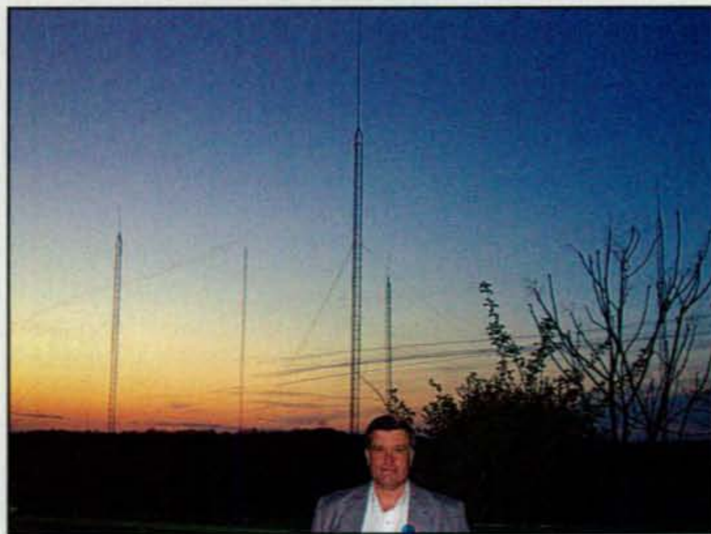
Pete, N0FW, with one of his 4-square antenna arrays. He has one each for 160 and 80 meters!
