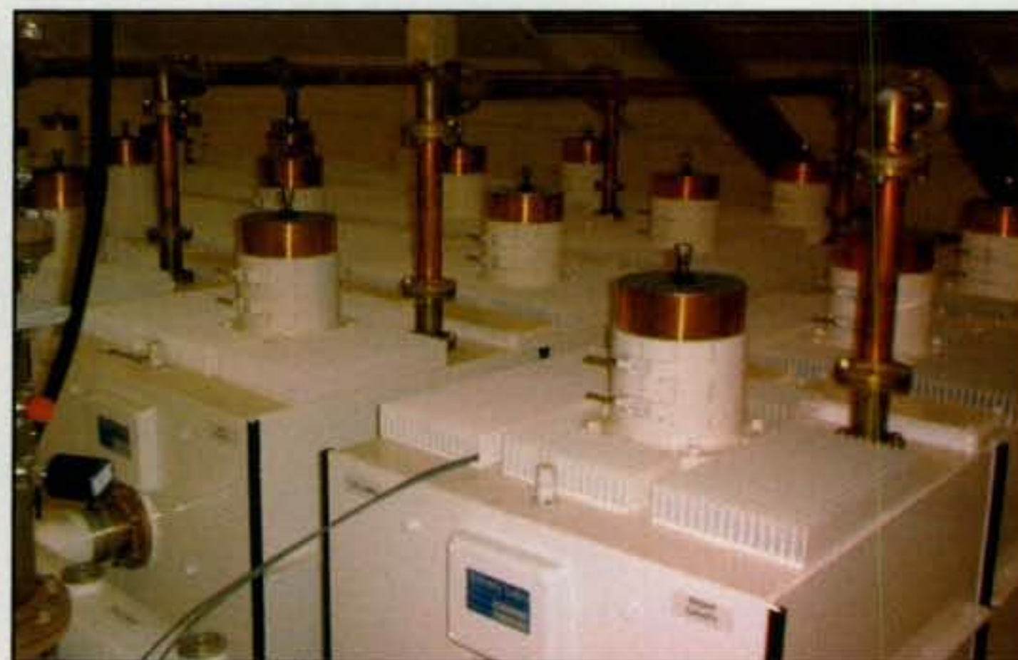
Photo D— Combining transmitters on the same frequency.
