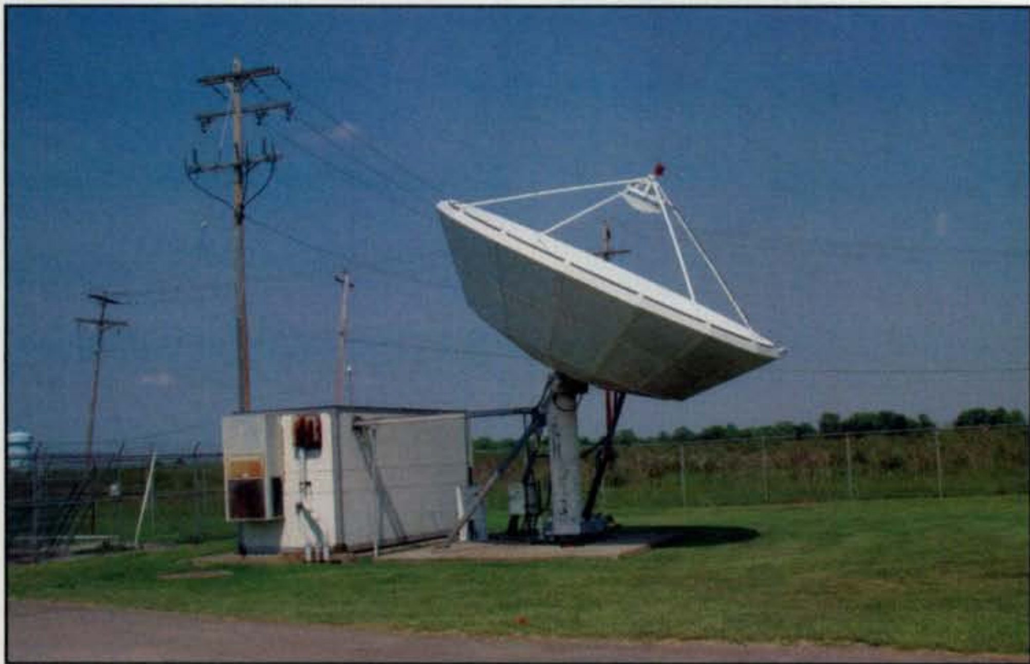
The 7.2-meter dish used for recent WC8VOA 10-GHz QSOs. (N6CL photo)
