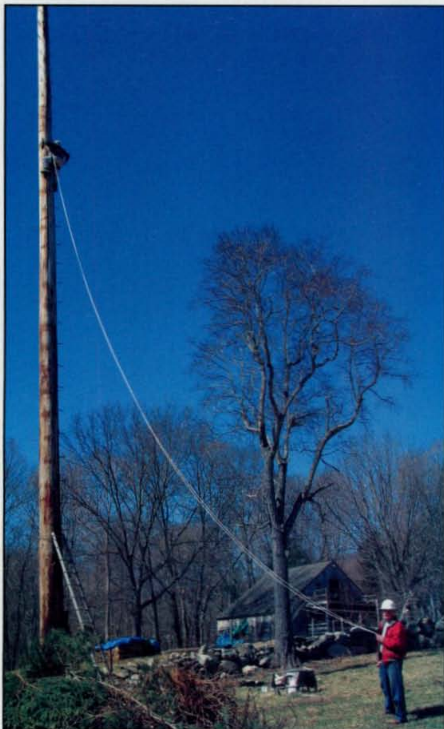
N2XN, wisely wearing a hardhat, holds my harness rope as I start patching one of the woodpecker holes.
