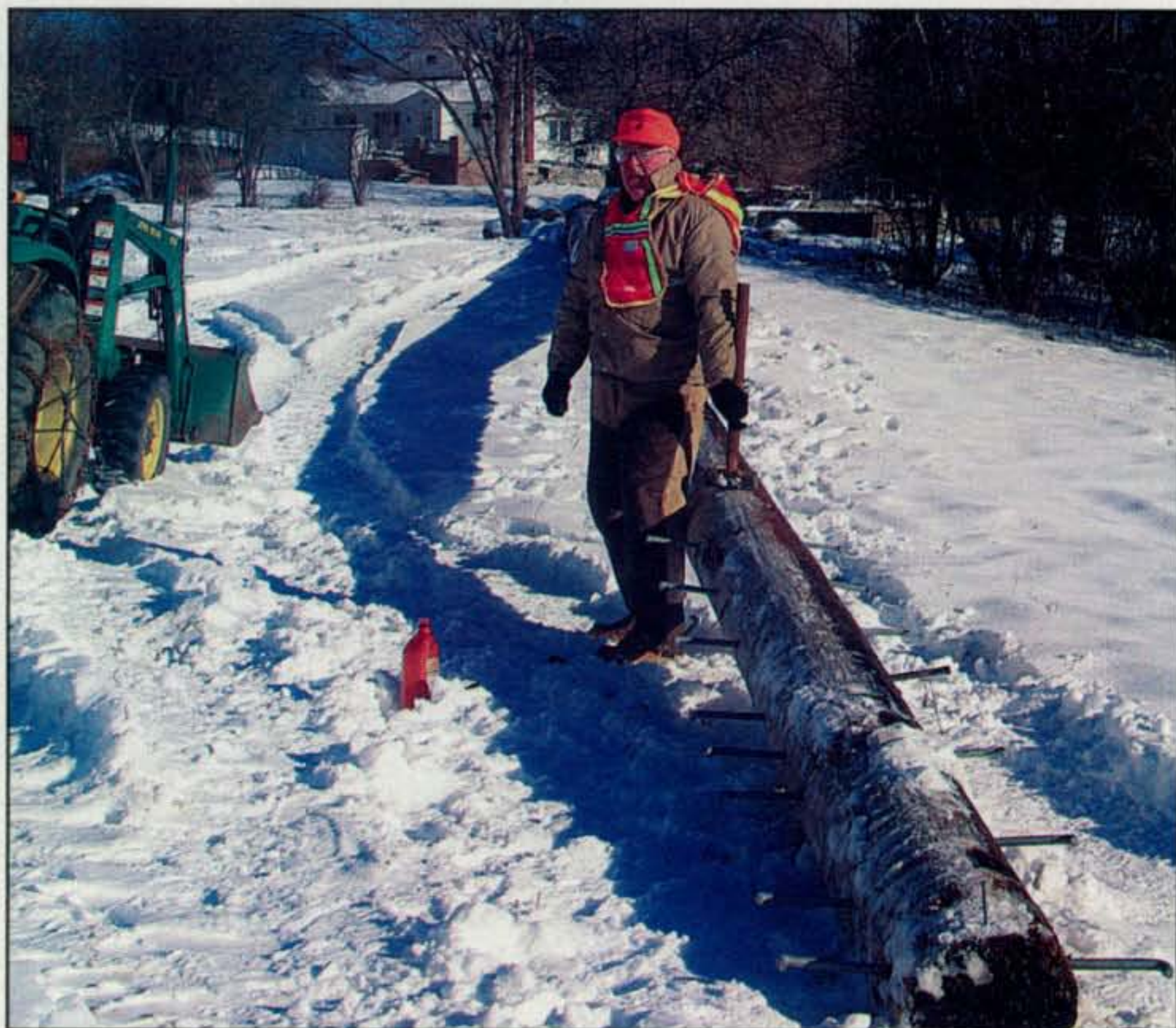
Setting the climbing spikes. I put them in every 12 inches and kind of spiraled them up the pole, since it is too wide for anyone to climb straight up.
