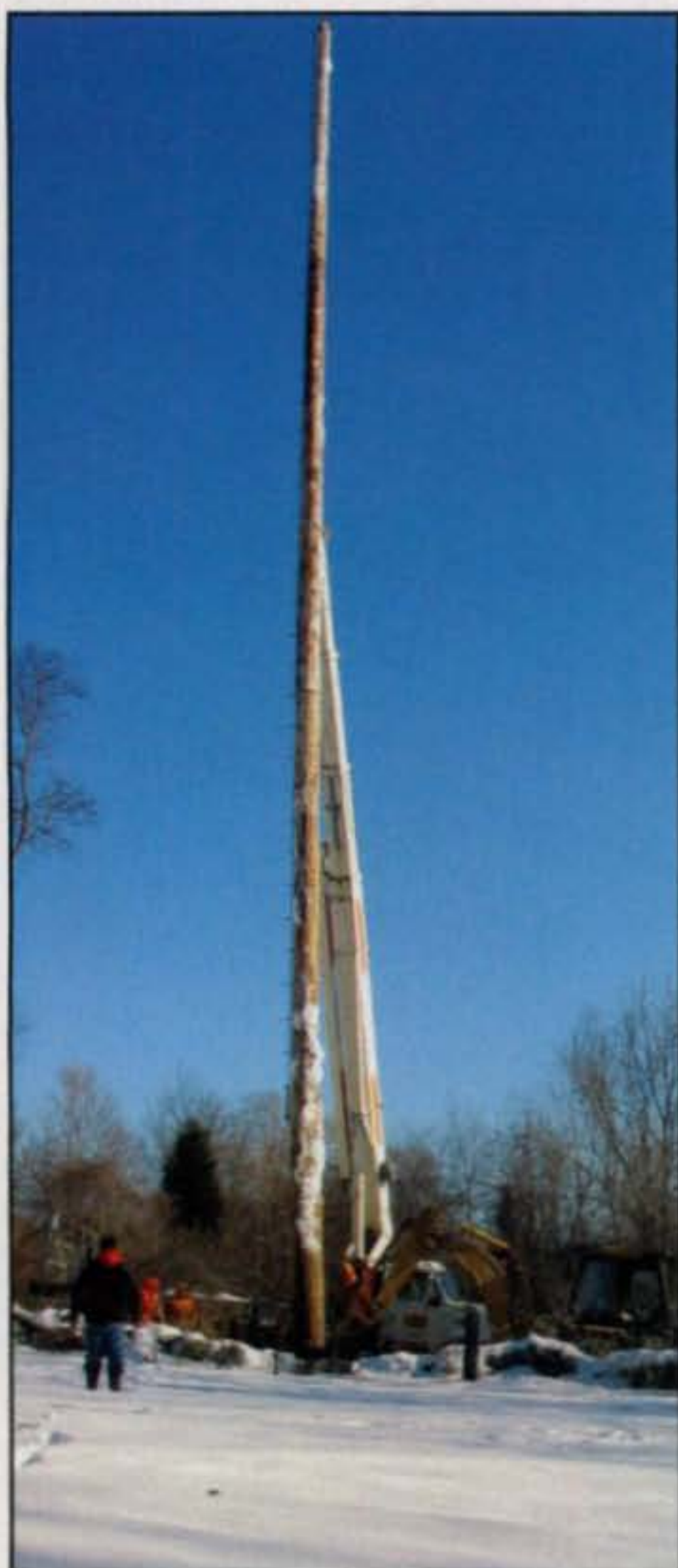
The pole, now in place, is admired from a distance.
