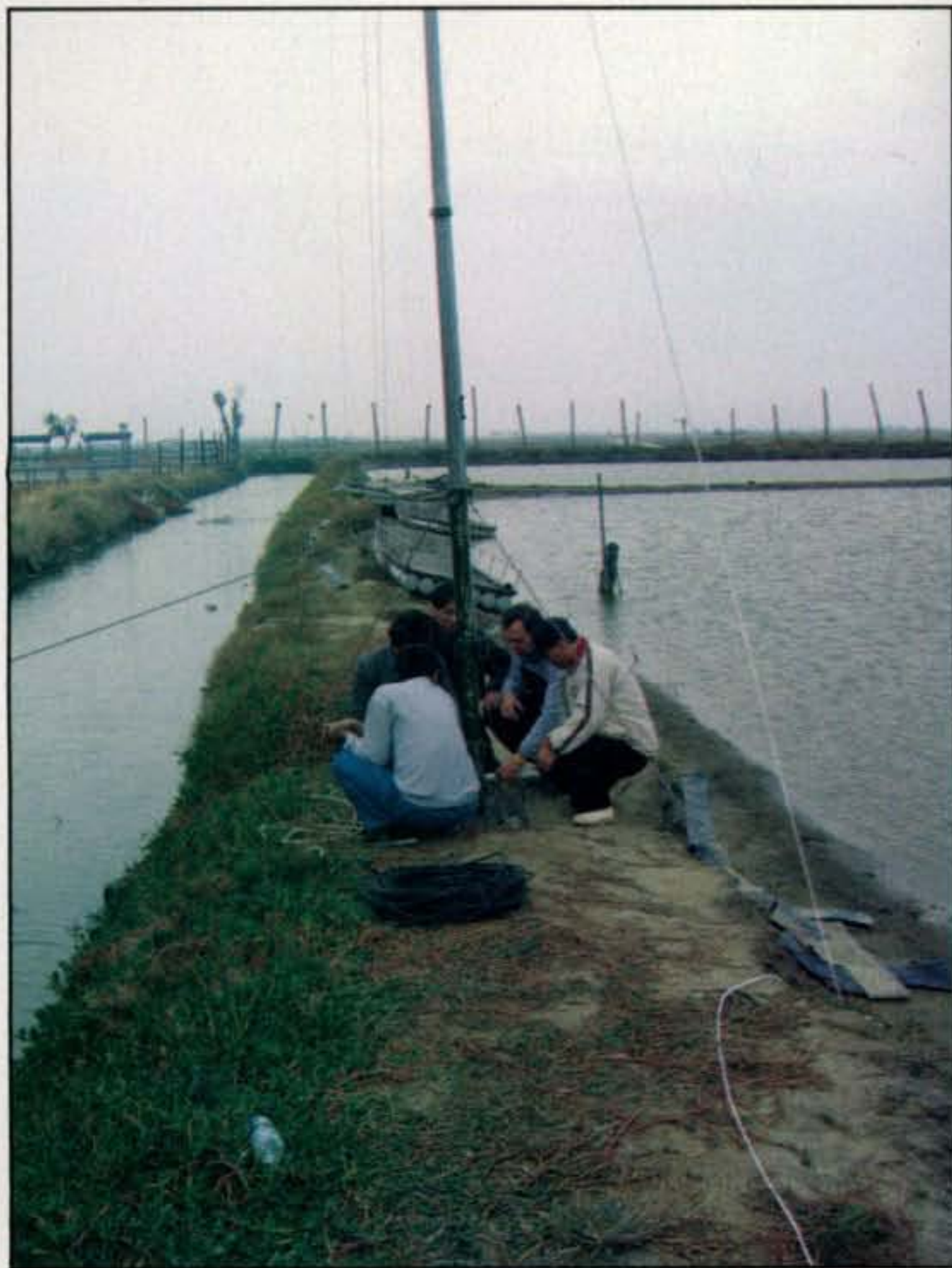
The 80-foot high Titanex 80/160-meter vertical, surrounded by salt water, was a superb transmitting antenna.
