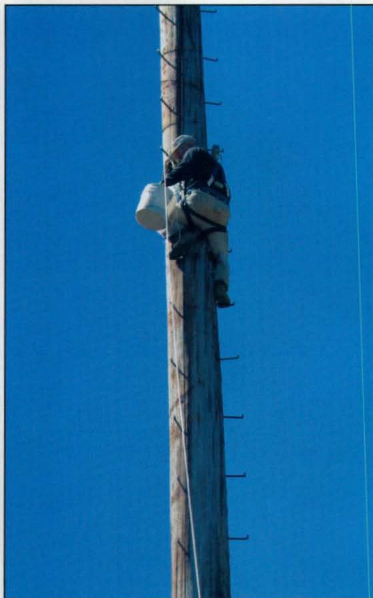
A bucket full of special epoxy was needed to patch the holes, but the woodpeckers came back and made new ones anyway!
