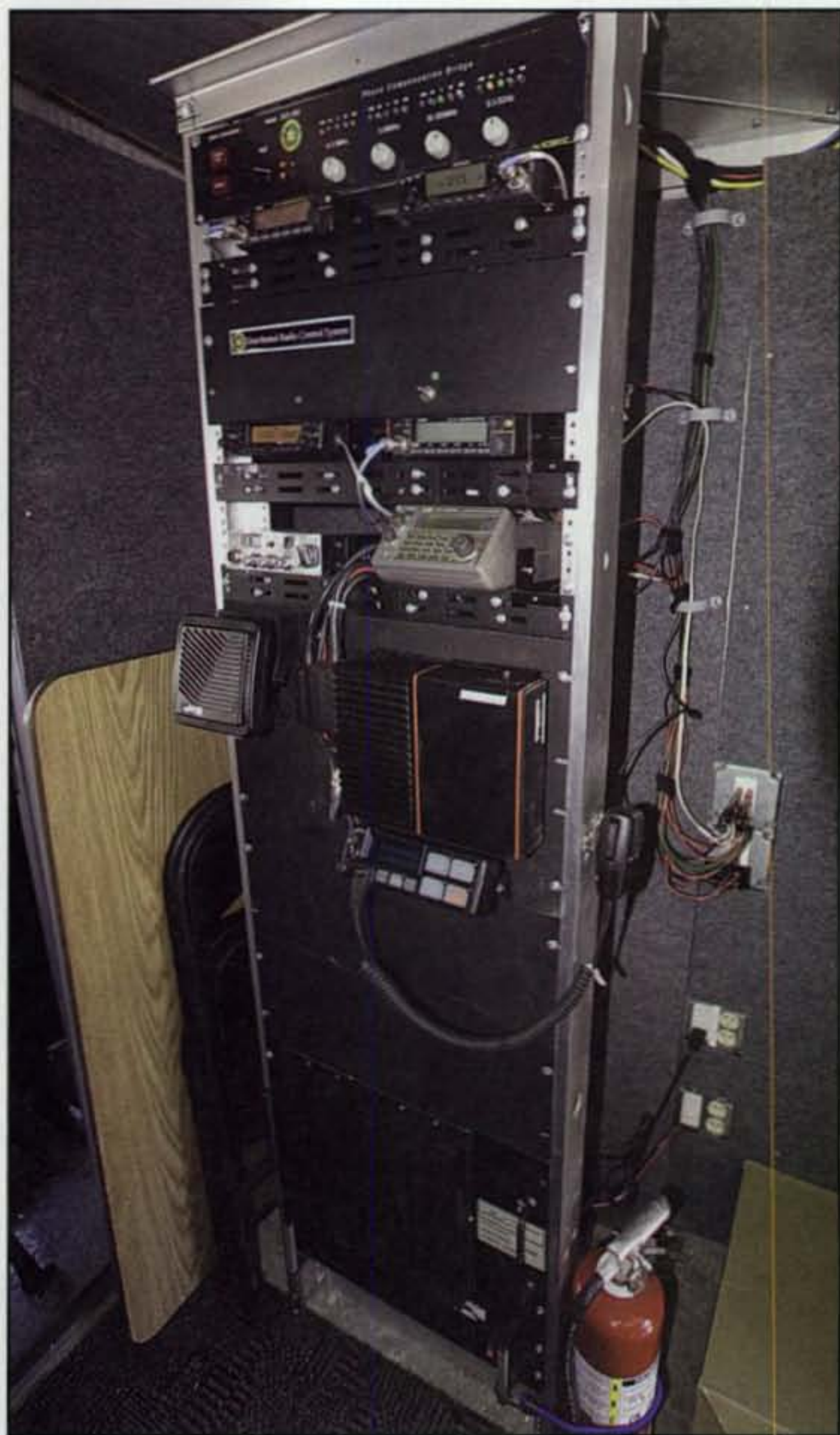
Radios are rack mounted for easy access and service, if needed.
