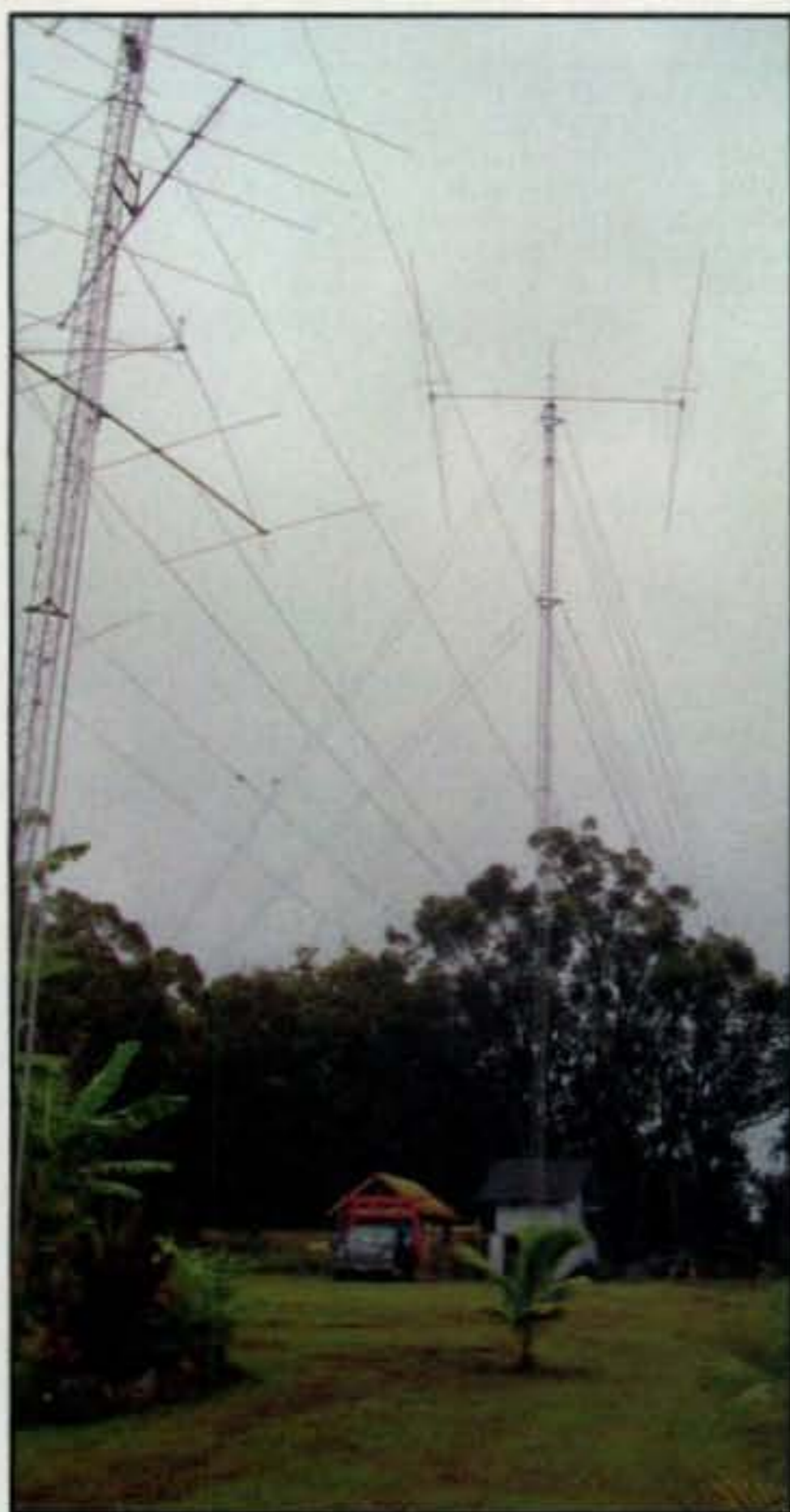
The tower in the center of this photo was rebuilt earlier this year and topped with a 3.5-MHz OptiBeam. Mike, KH6ND, says this is the site of former KH6XX and KH7R operations. It now belongs to Alex, KH6YY. Look out for some big signals this contest season. (Photo courtesy of KH6ND)
