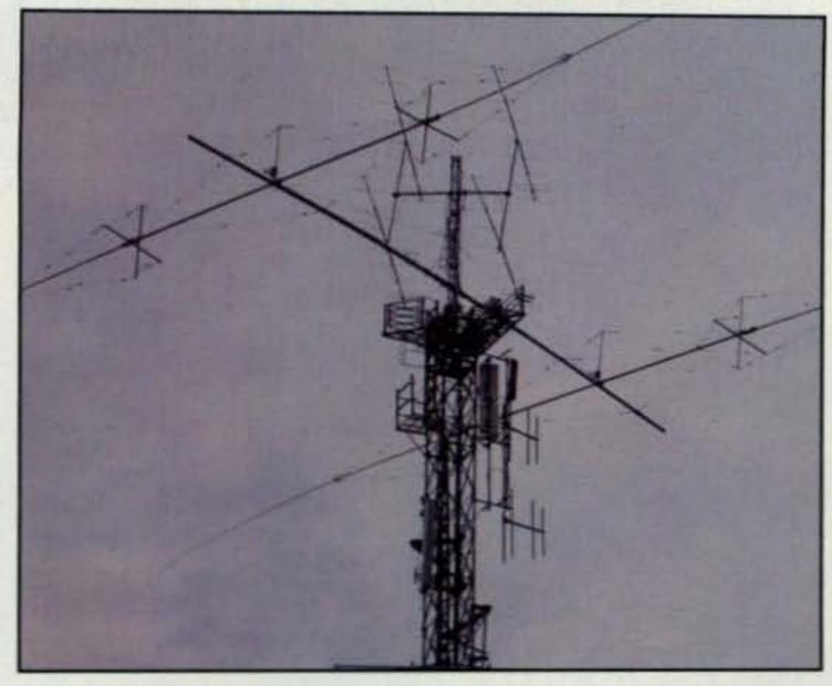
YT6A's full-size 80-meter beam made us very loud on 3.5 MHz!
