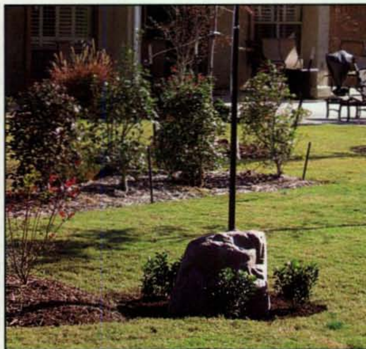
Photo 2— An up-close view of Bob’s “magic rock” that, as discussed in the text, is a decorative fiberglass enclosure sold to hide outdoor faucets, etc. Bob cut a hole in the fiberglass to pass the vertical through and added small shrubs to produce a neat, natural-looking landscape. The transmission line to the house 40 feet away is also buried.
