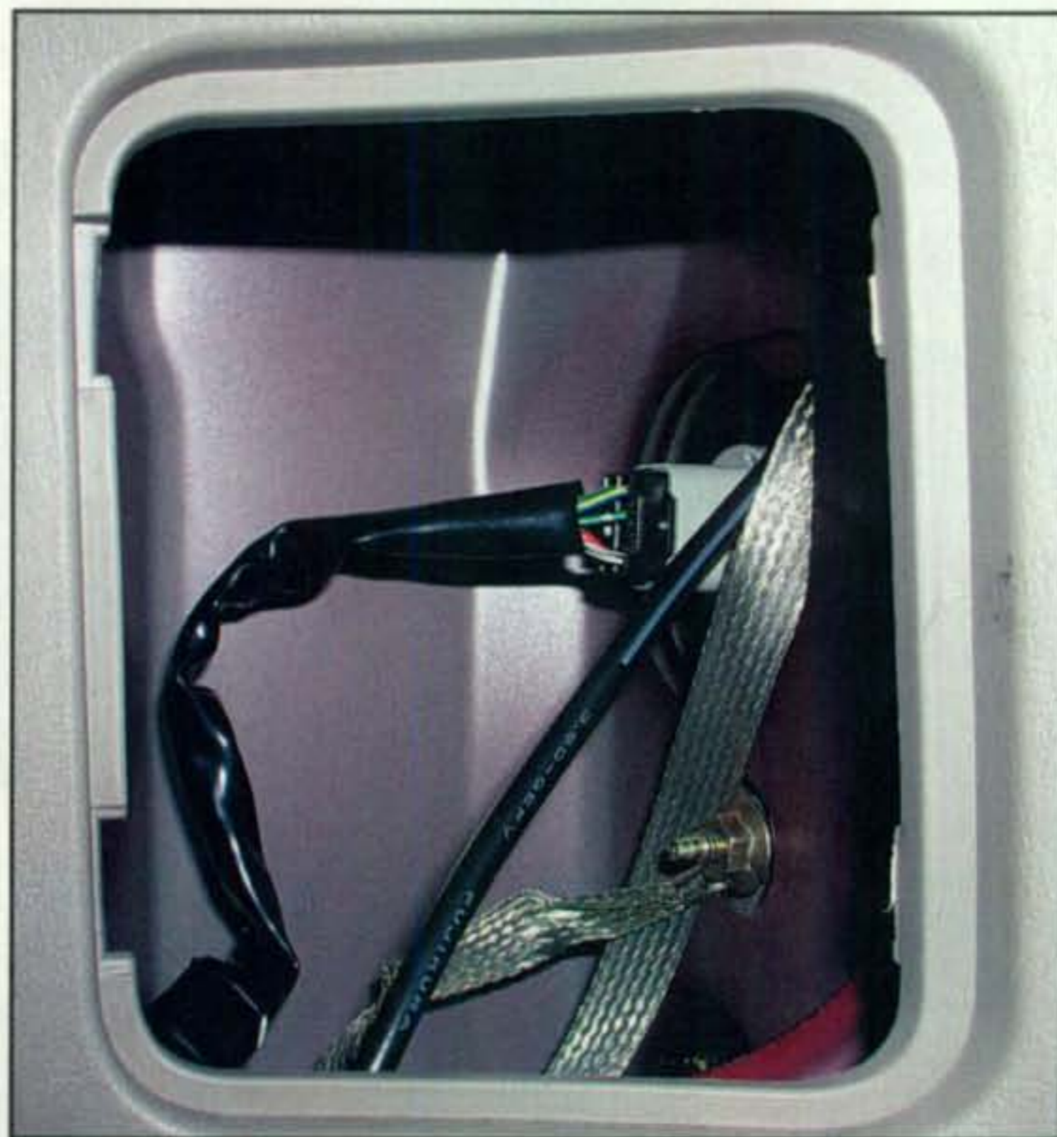
Detail on how the coax and ground braid were routed into the SUV and the secure ground connection, making a weather-proof contact with the vehicle's body.
