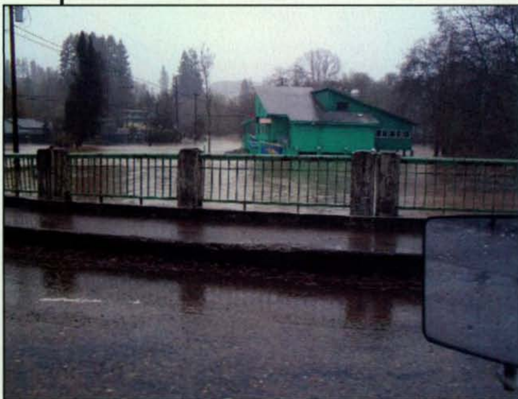
Residents were evacuated from the hard-hit town of Vernonia, Oregon as the Nehalem River overflowed its banks. (Photo courtesy of Reo Gargovich, KE7REO)
