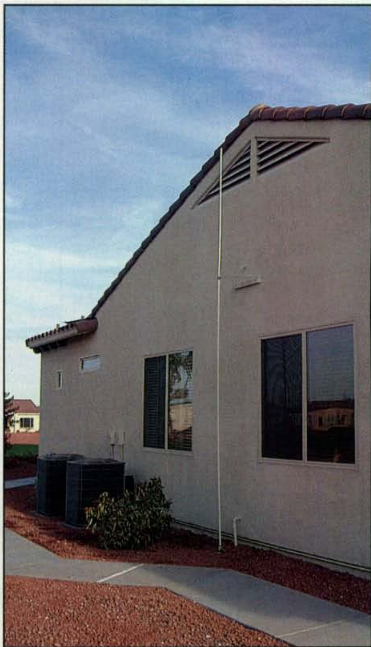
Photo B— A closer view of the 17-foot tall AD7JT 20-meter vertical. Painting antenna elements for camouflaging does not degrade performance, provided the paint does not contain lead or metal. Krylon® paint works very well. This antenna is so low profile it could easily be mistaken for an overflow drain for an attic-located water heater. (Photo courtesy of AD7JT)
