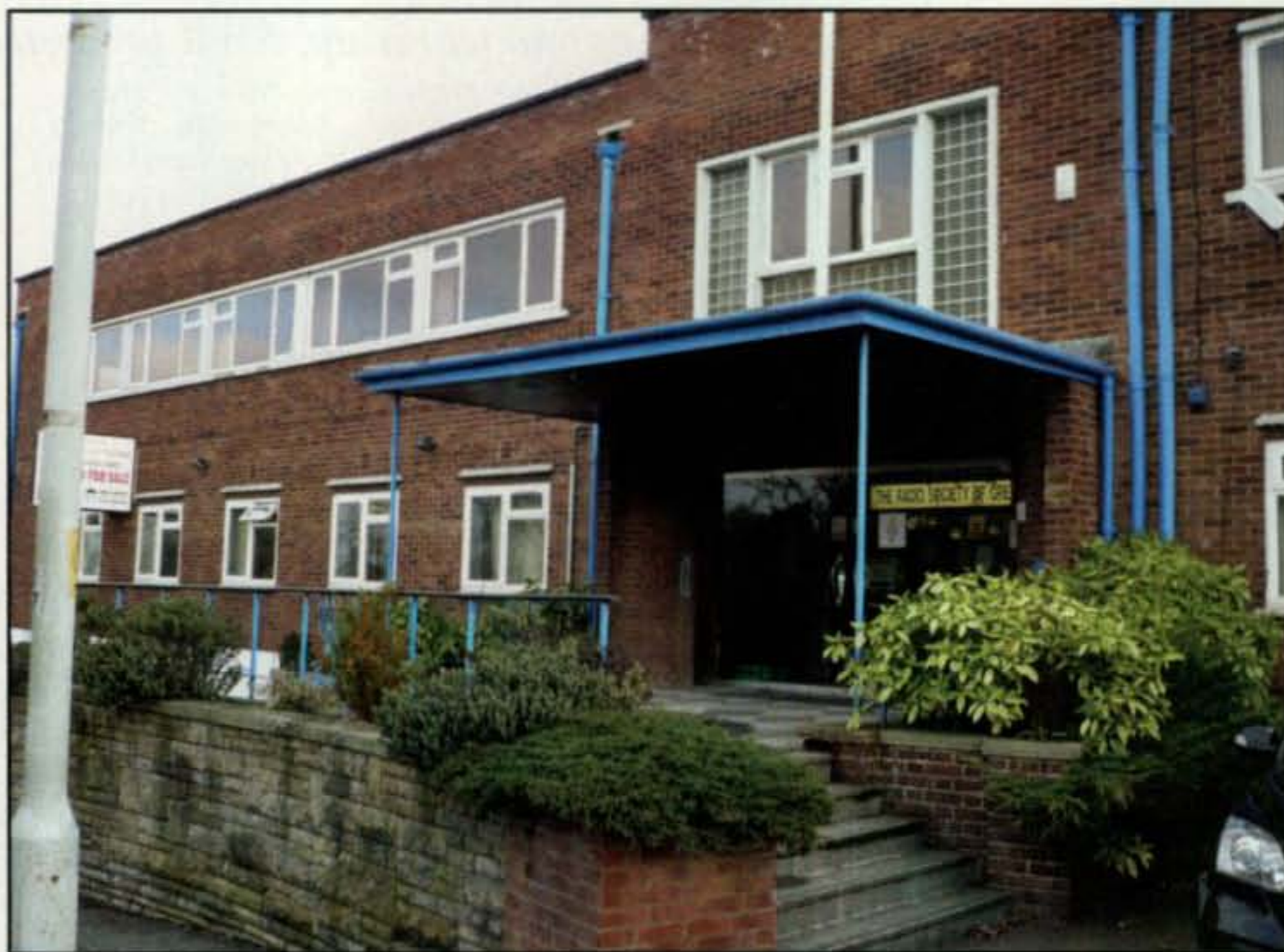
Photo A— The Radio Society of Great Britain's (former) headquarters building, Lambda House, in Potters Bar, north of London. (All photos courtesy of the author)
