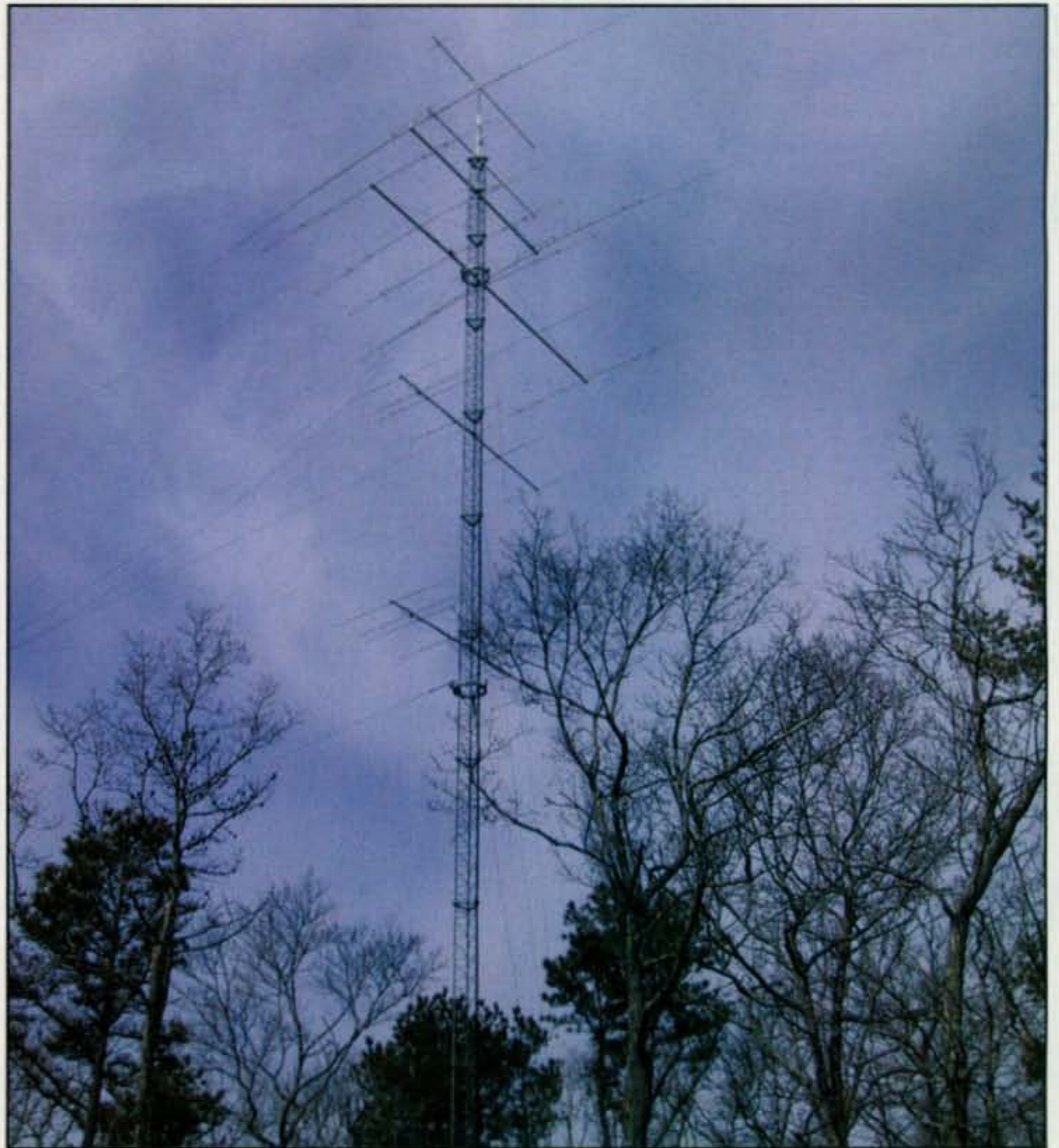
Fig. 1— The author's 100-ft. rotating tower, the subject of this article. Majestic, isn't it? (Photo by KB1LN)
