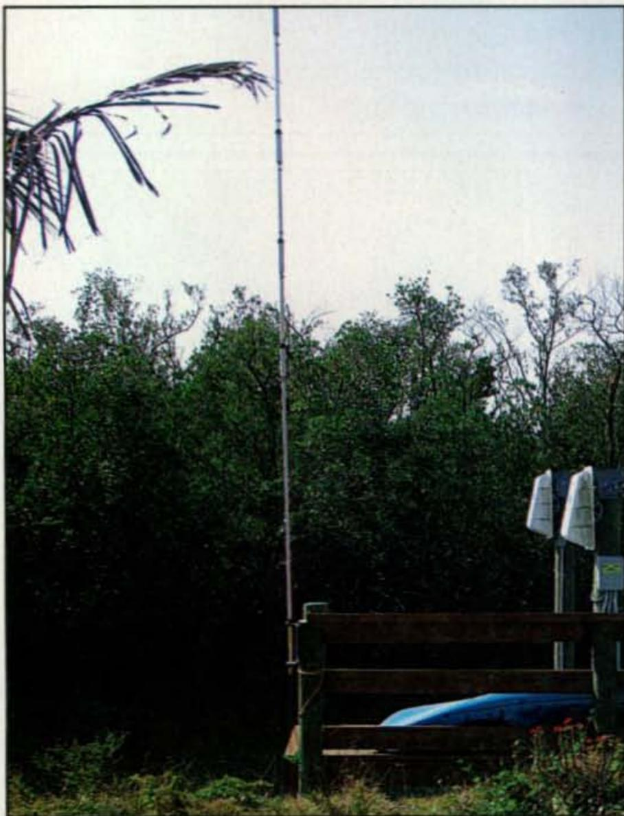
Photo A— During a recent QRP QSO with Alan, W4MQC, I asked about his rig and antenna, and he shared this photo. Alan uses a Hustler 6BTV Vertical mounted to the boat dock behind his house. A single radial routes down the piling and into the salt water, which is highly conductive and goes right into the Gulf of Mexico. Now that's a big-time ground system for sure!
