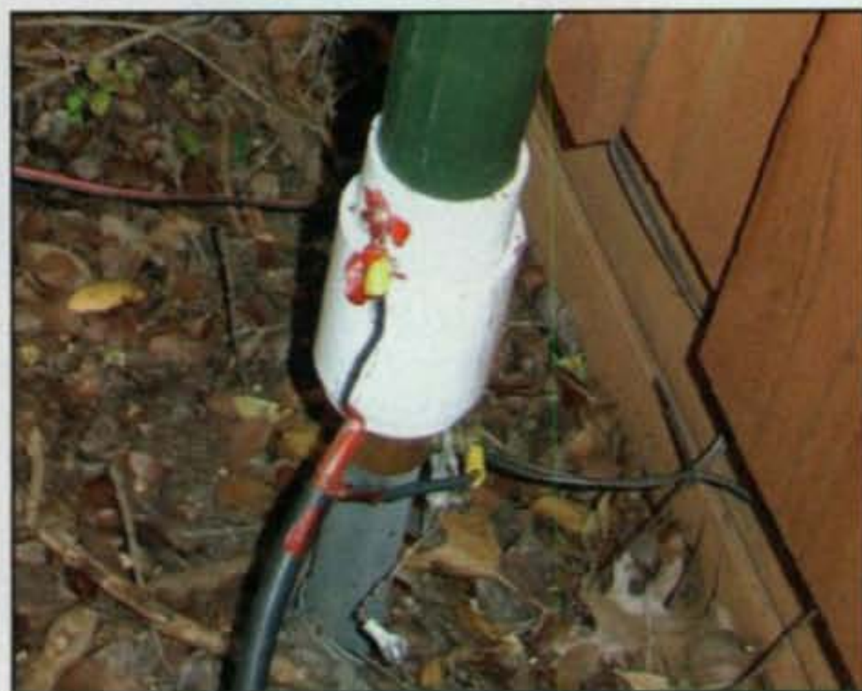
Photo D— PVC insulator at the antenna base.
