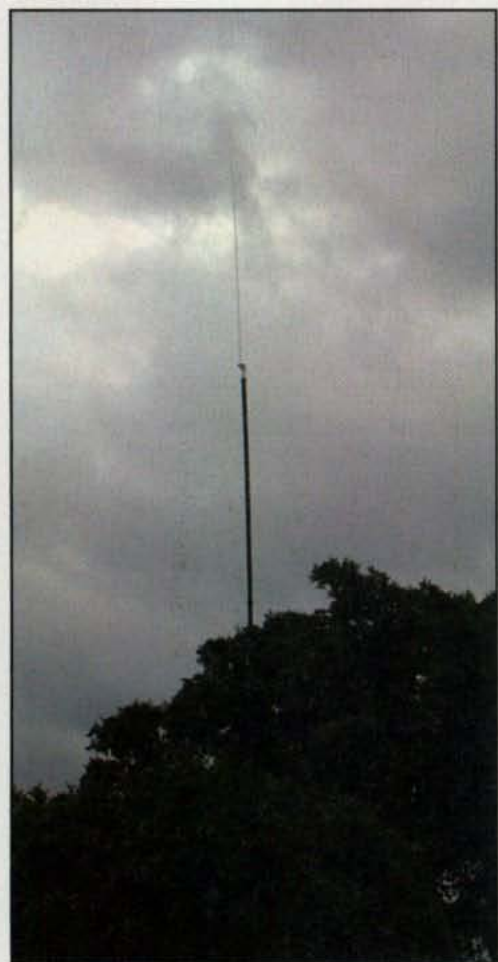
Photo F— Distant view of the antenna.
