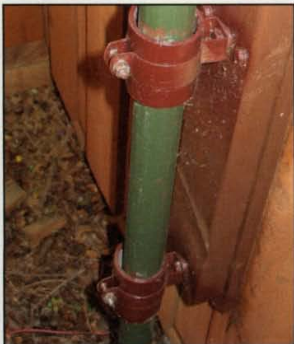
Photo E— Two-inch PVC and fence mounting brackets support the antenna. The PVC was painted brown to match the fence color.
