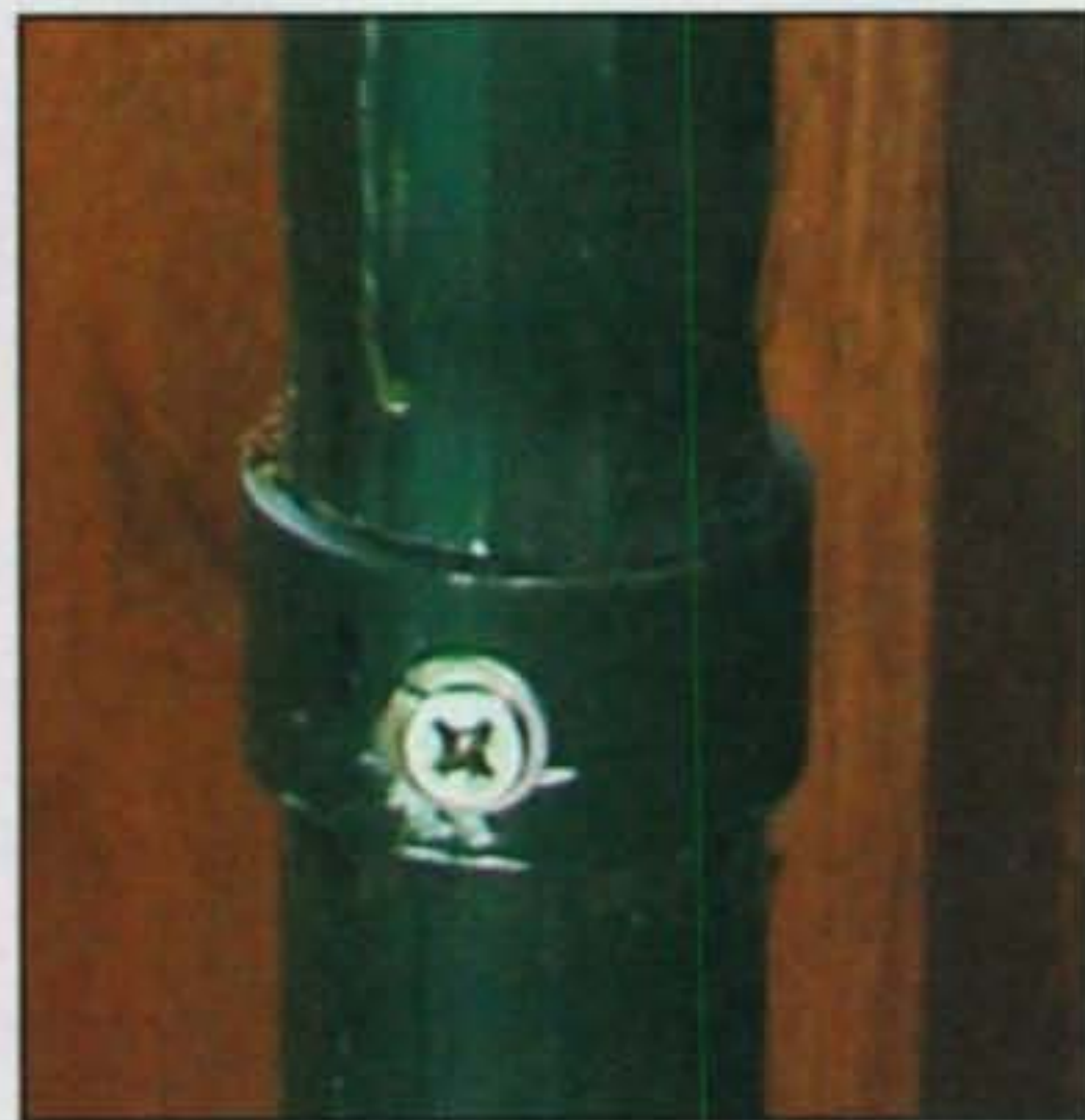
Photo B— No. 8 screws used to lock the aluminum sections together.
