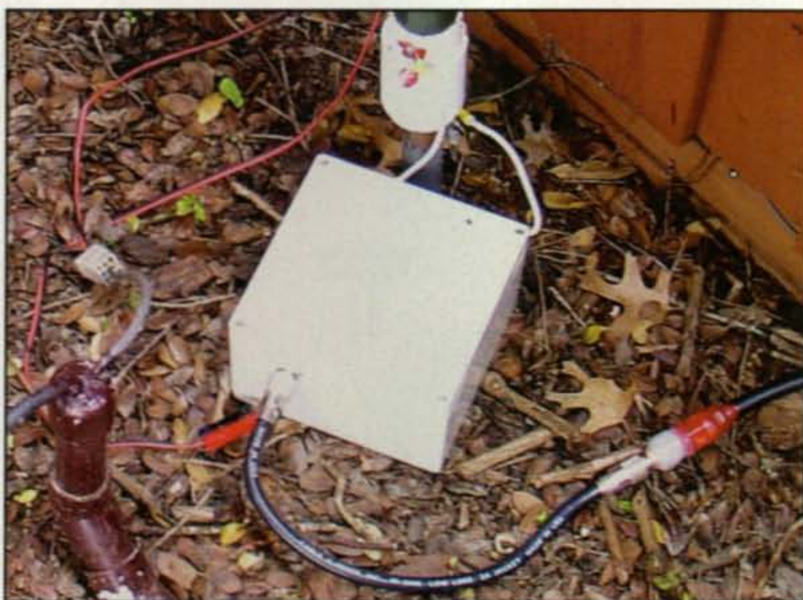
Photo B— Matchbox installed at the 36-foot vertical antenna base.
