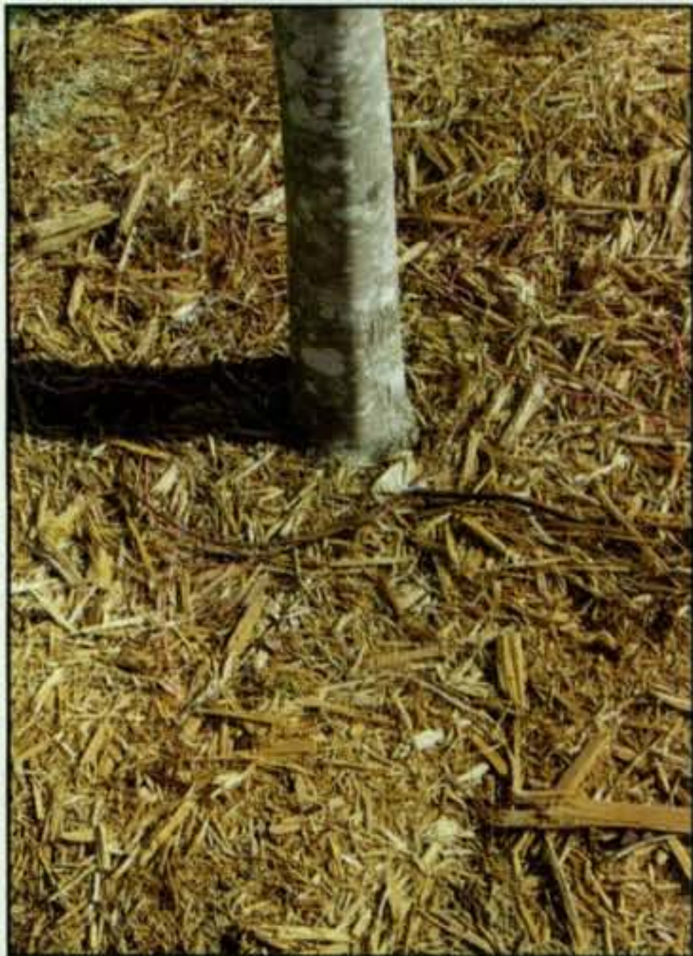
Photo B—Close-up view of the tree base supporting three antennas at N6SL. All three radiators are parallel-connected to the single coax feed line's center conductor, and 10 buried radials are parallel-connected to the feed line's shield. Even in direct sunlight the wires and cables are barely noticeable (especially with the pine-bark distraction), and that is precisely the objective.
