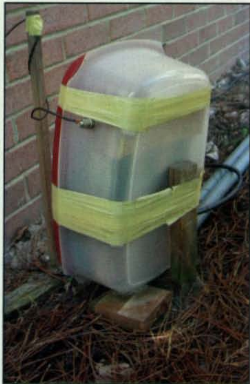
Photo 4— RF feedpoint of the K8CQ "Gutter Tenna." Transmission line from the indoor station connects to a SGC-237 tuner in a weatherproof plastic box. Output wire from tuner is attached to the base of the downspout with a sheet metal screw. Since the antenna is low and close to the living area, Jeff never uses over 100 watts of power. (Photo courtesy K8CQ)
