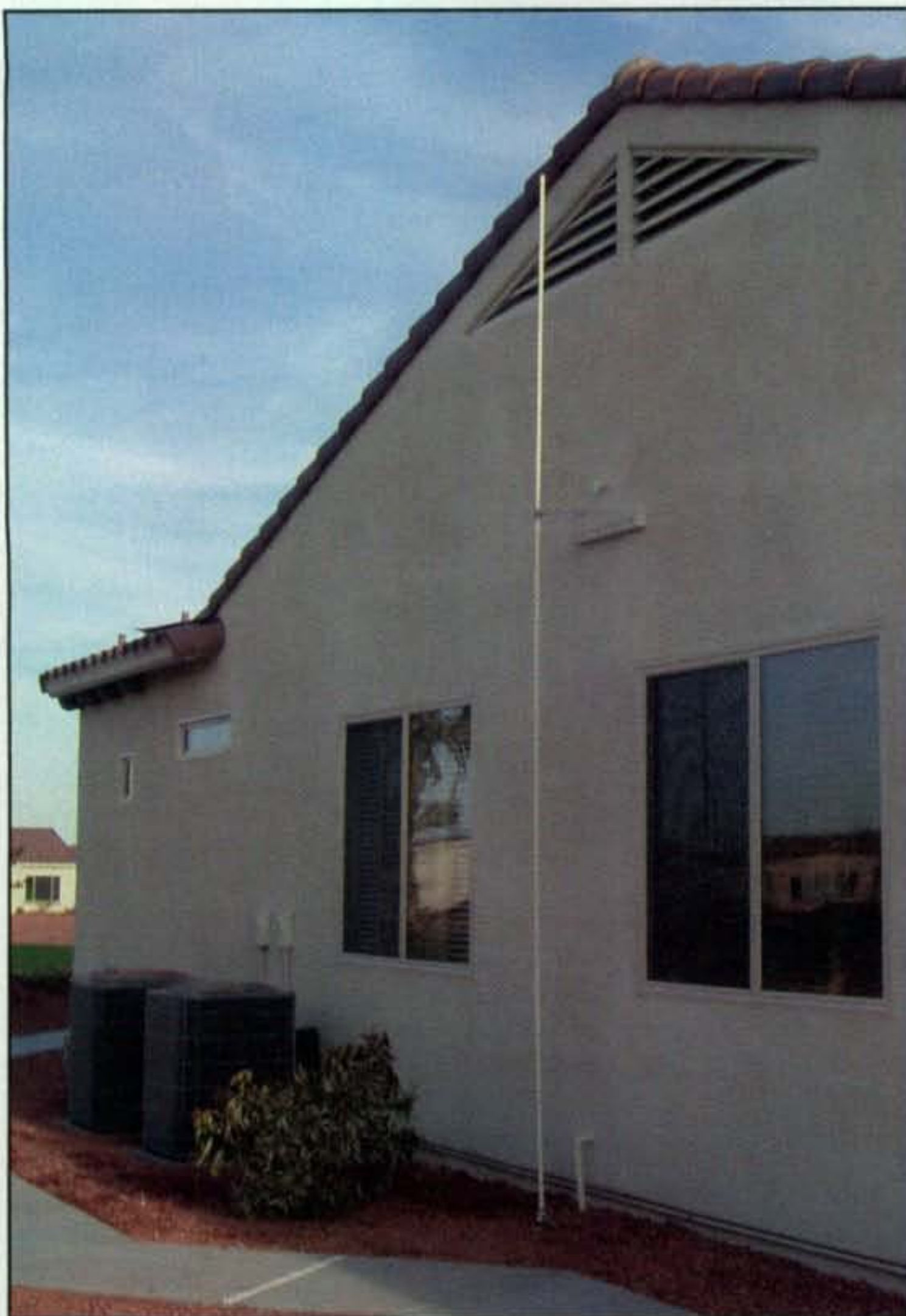
Photo 6— Is that a drain pipe for an attic-mounted water heater beside the house of AD7JT? No, it is a painted-to-match 20-meter vertical antenna. It could, however, be changed to a SteppIR vertical modified for gain-type 3/8 -wave operation as discussed in the text. Add a plastic reflector and phony light to the top, and it could even pass as an emergency night light to foil prowlers.
