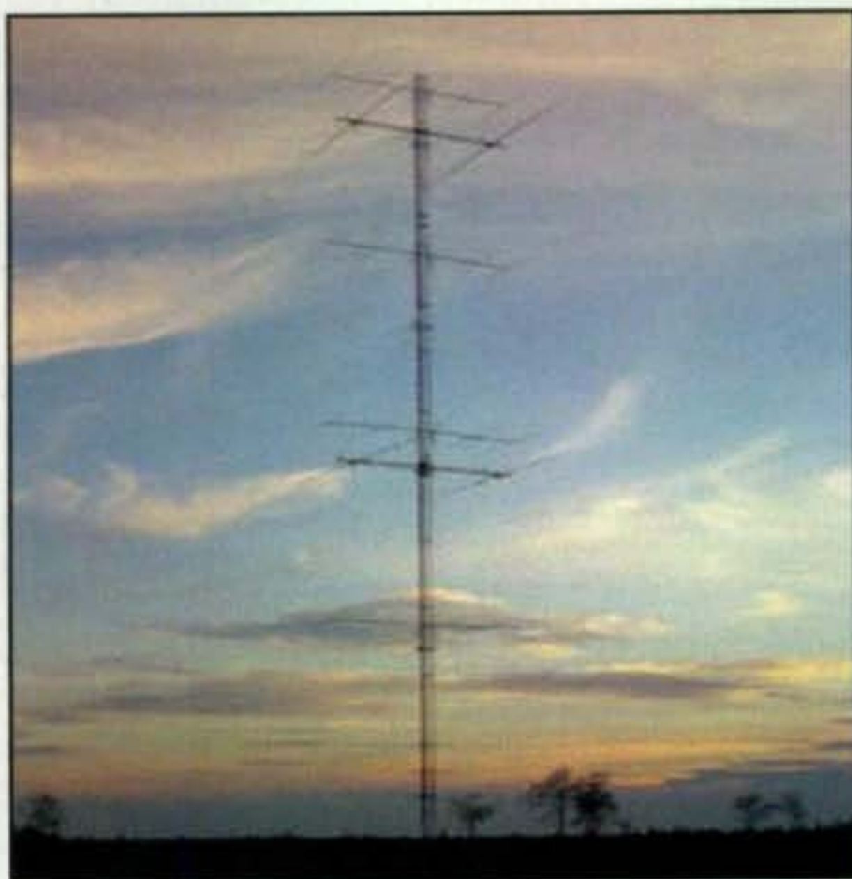
OH8X 300-foot tower with four 6-element 20-meter stack and 2 over 2 for 80. (Photo from the OH8X website)
