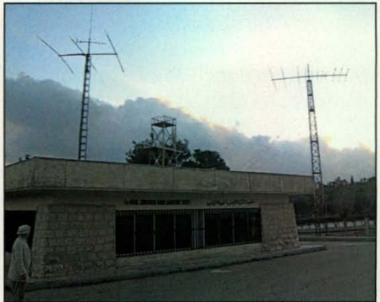
Photo D— The Royal Jordanian Radio Amateurs Society building and antennas for club station JY6ZZ.
