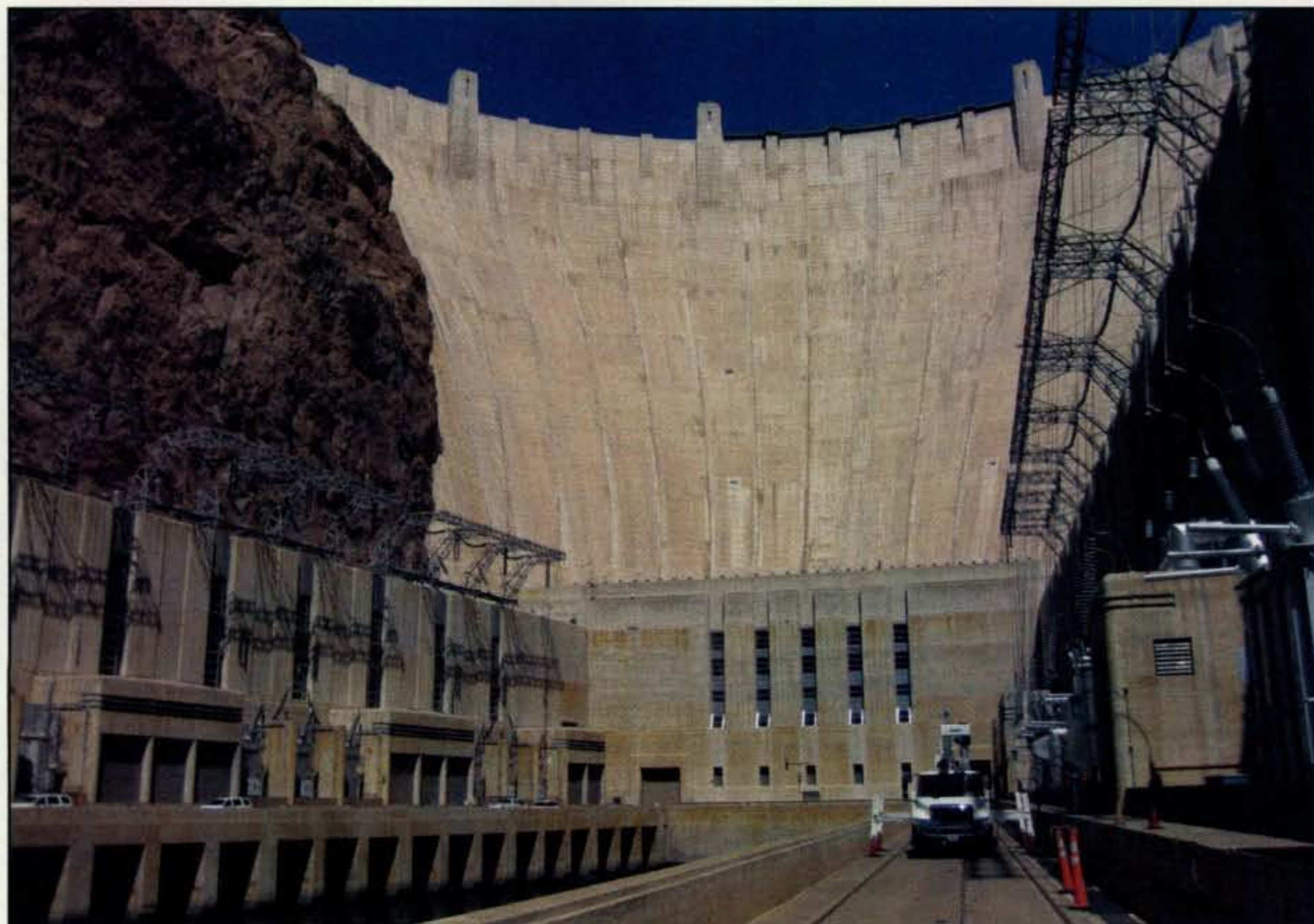
A rare look at Hoover Dam from its base, holding back the contents of Lake Mead through its sheer mass and providing a home to 17 powerful generators. (All photos by the author)
