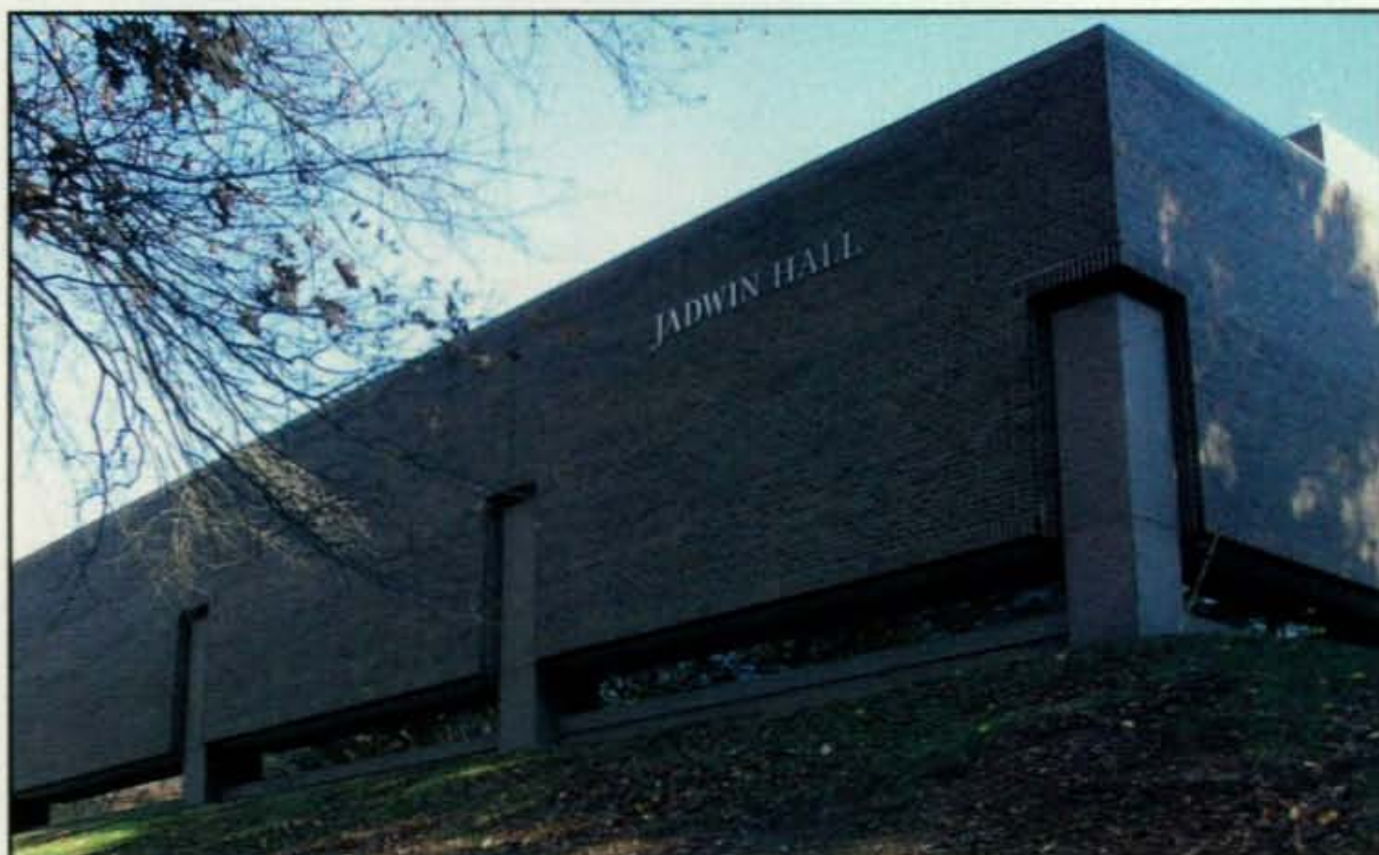
Jadwin Hall is home to Princeton University's Physics Department. It was built into a hillside to insulate basement laboratories from street vibrations.
