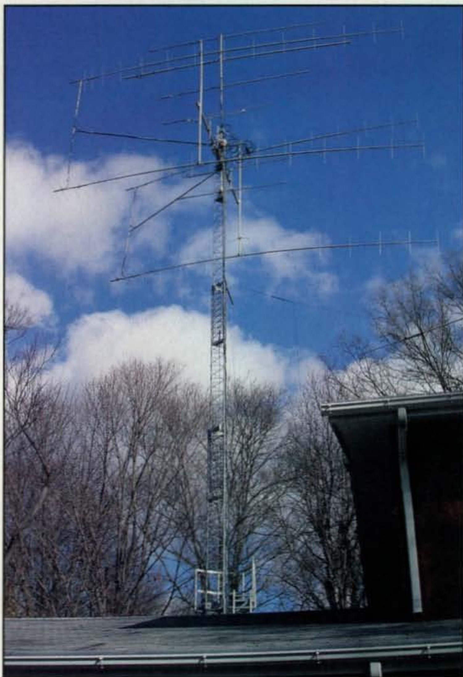
Joe's 70-foot back-yard tower is dominated by his 2-meter EME array—not surprising for someone who revolutionized amateur moonbounce communications. See the sidebar "At Home with K1JT" for descriptions of all of the antennas on the tower.
