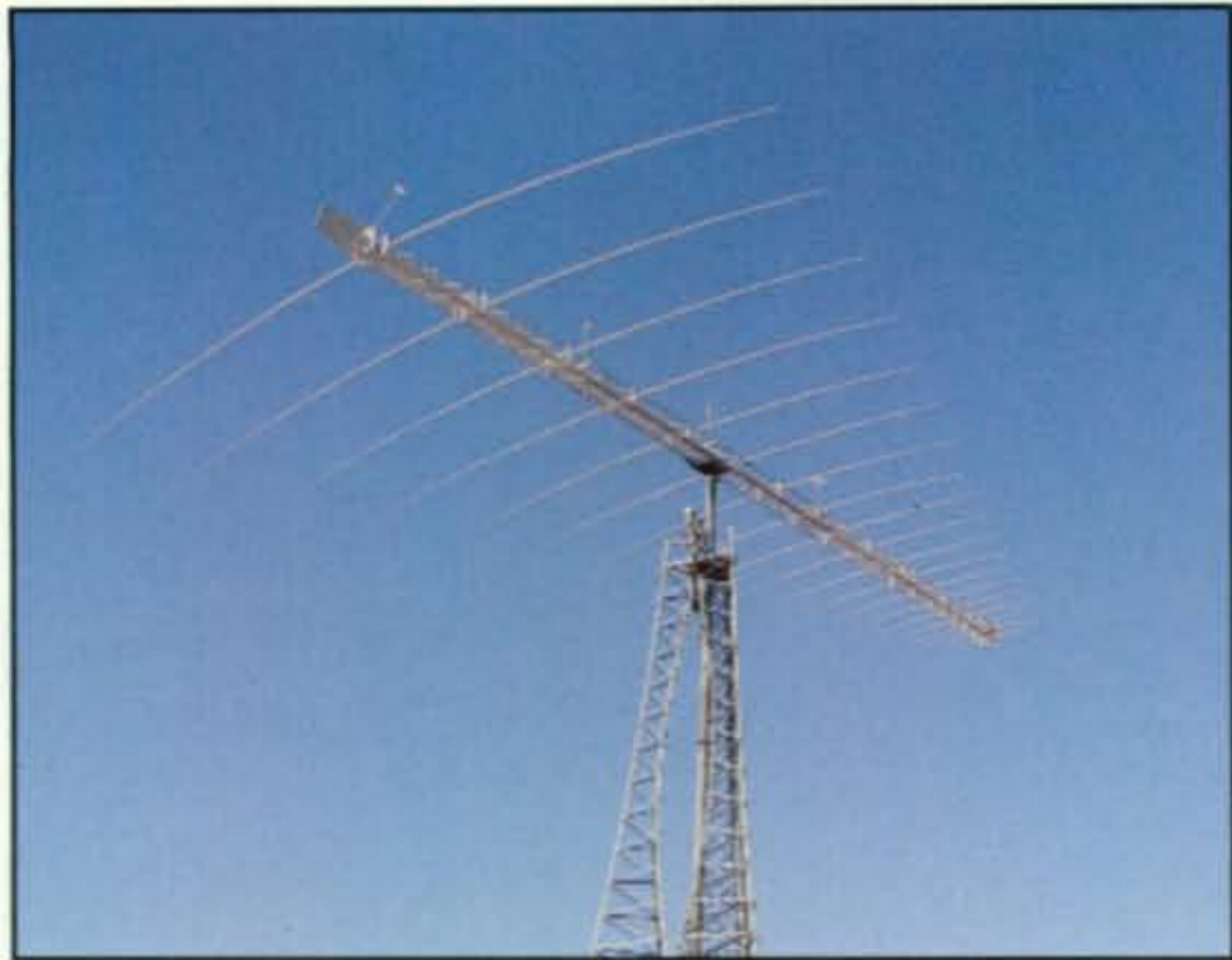
Log-periodic antennas are becoming very popular. Here is a monster going up at N5WV. It has 19 elements covering 5 to 30 MHz and will be installed at 200 feet. (Photo courtesy of Randy, N5WV)
