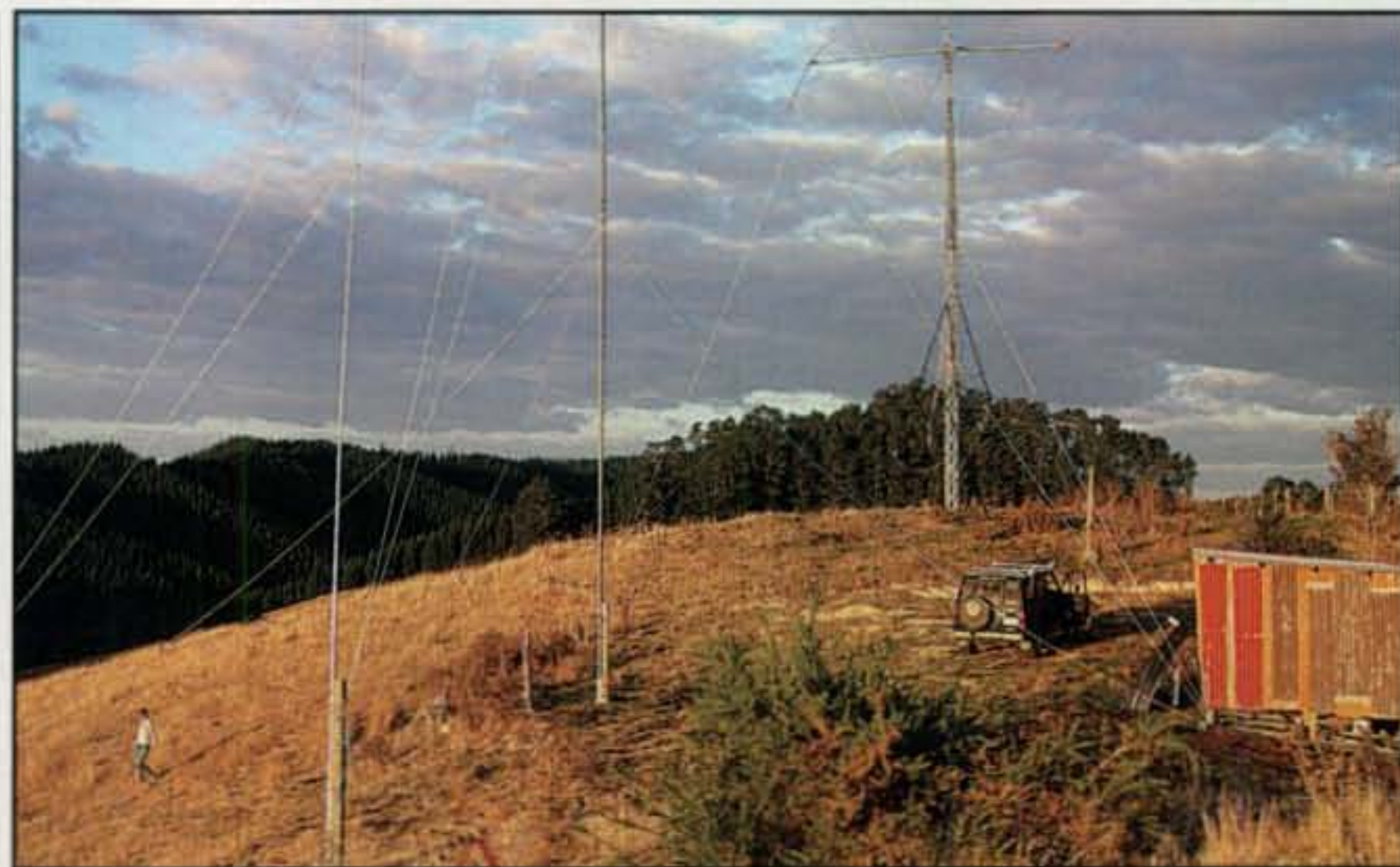
The antenna field at ZM3A, world high score for 40-meter single band. The 3-element Yagi can crank up to 24 meters above a very nice hilltop location.
