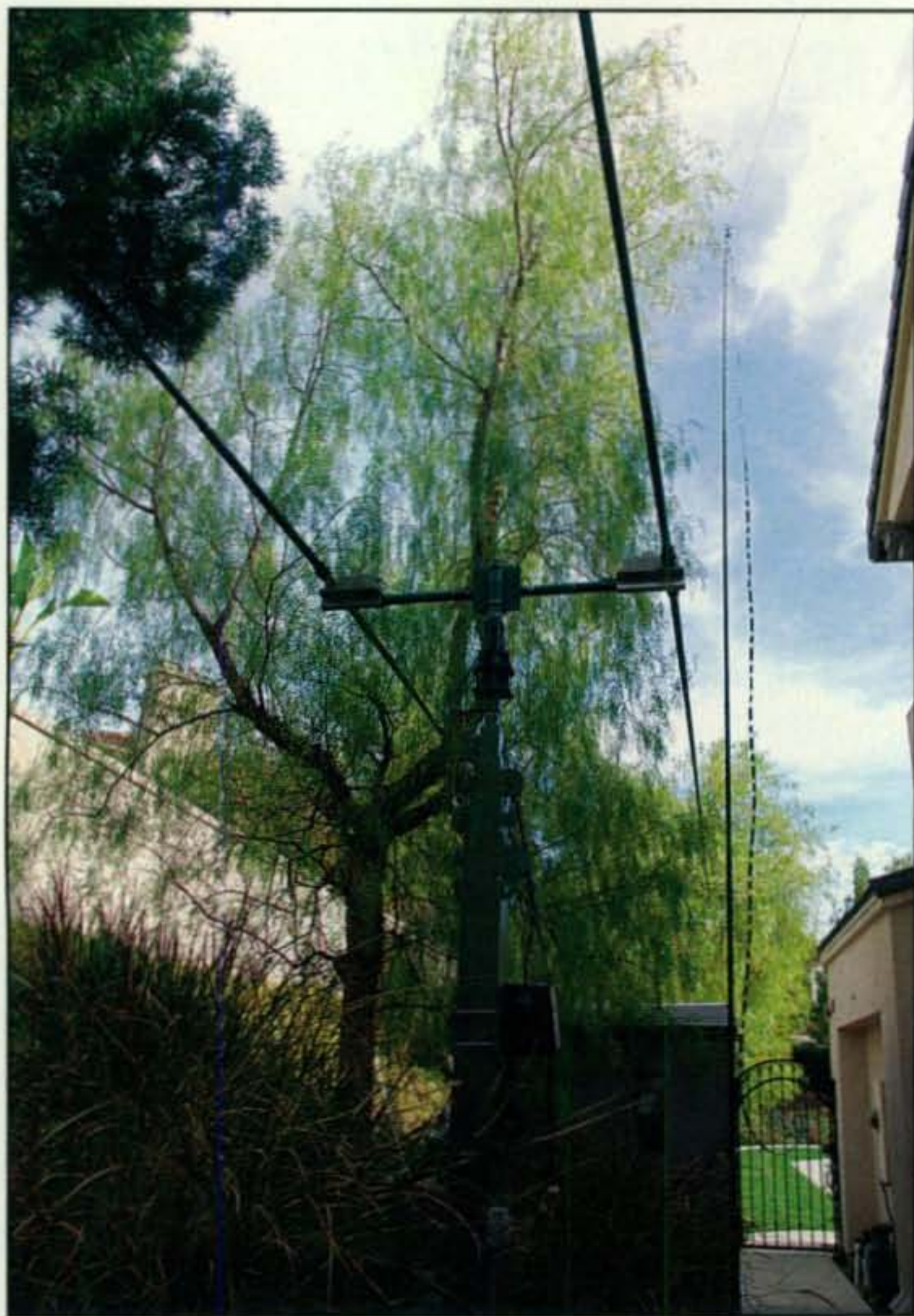
Photo C—A first view of the hidden antenna farm at QTH of Howard Hawkins, K6BYU. The 2-element SteppIR beam with olive-green elements and boom plus motorized tower, also painted green, is lowered and nesting in foliage while 32-foot pole supporting a G5RV is raised. All antennas are behind the house and inside gated yard. (Photo courtesy of K6BYU)
