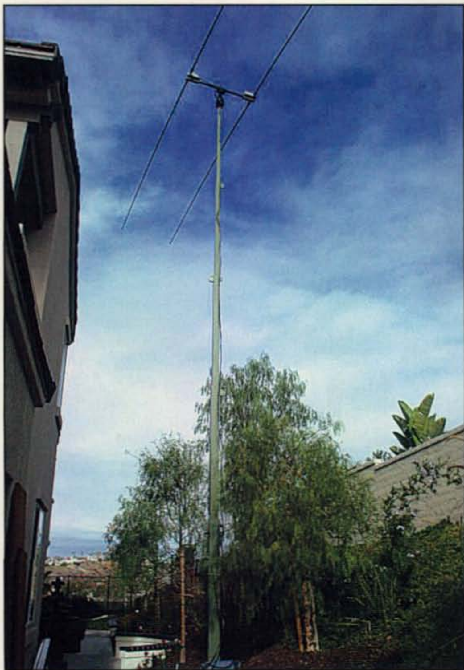
Photo E— A couple of minutes later, the SteppIR beam has been raised to nearly 50 feet (magnificent little gem, isn't it?) and the 32-foot vertical has been tilted down out of sight.
