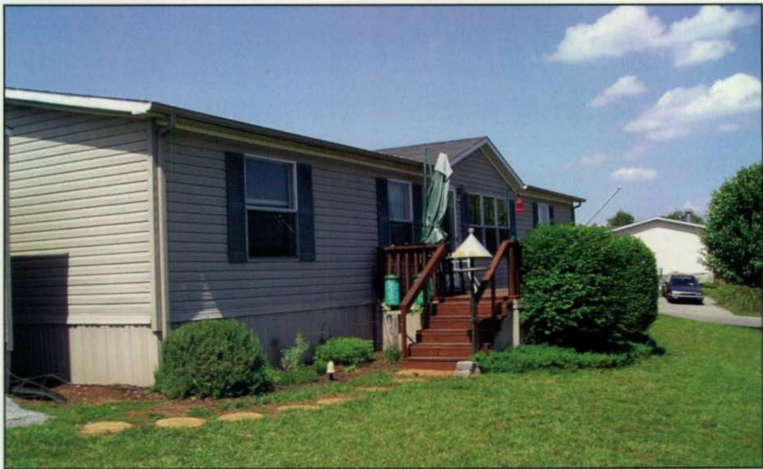
Photo A— Can you spot the multiband antenna at this QTH of Dave Winkle, WA8KOQ? Neither can suspicious eyes. It is comprised of dual rain gutters on each side of the house front, with a white-insulated wire attached to the eaves of the peaked section, connecting the sides. An auto tuner is located out of view at the feedpoint, which is at base of the downspout. Photo courtesy of WA8KOQ)
